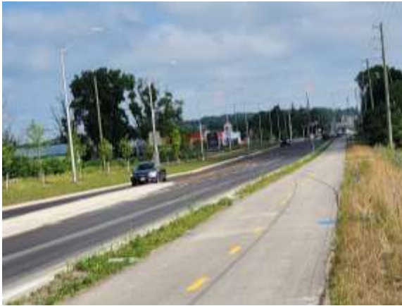
View to north of Colonel Talbot Rd, adjacent to Ph. 1
