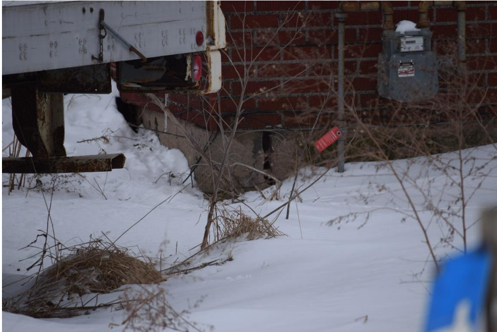
Photo 7: Parged foundation, looking south
