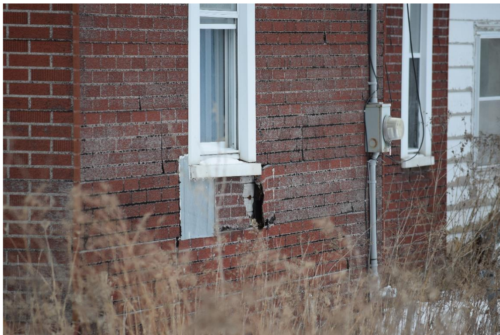
Photo 6: Asphalt brick siding on west façade, looking shingles
