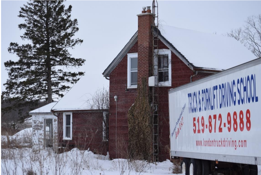
Photo 9: East façade, looking southwest
