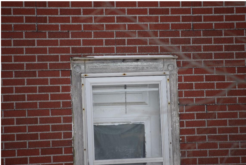
Photo 8: Wood door surround, looking south
