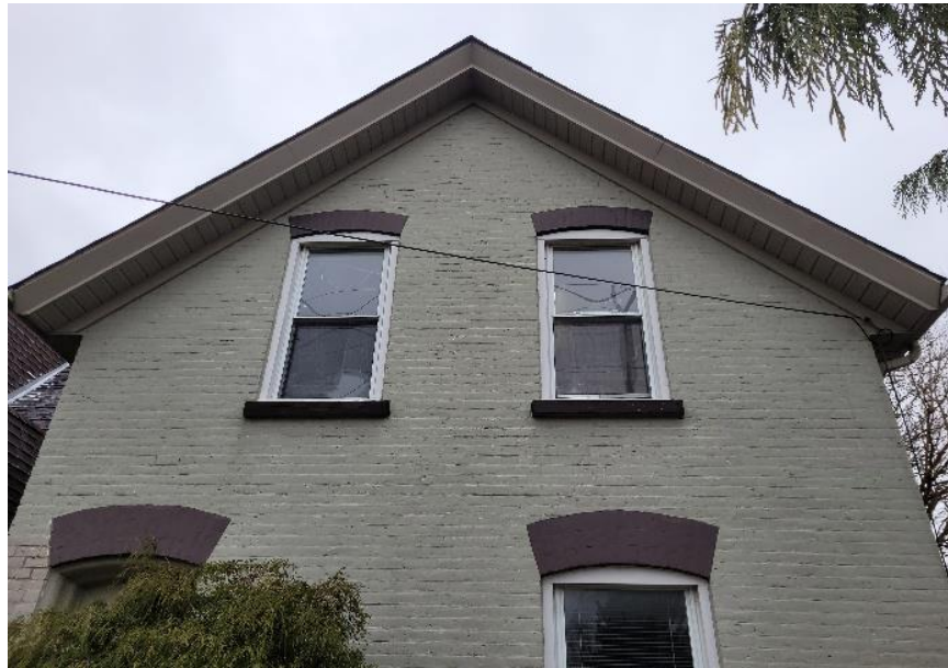
Photograph 14: View of the second storey windows on west wing of the north elevation (AECOM, 2025)
