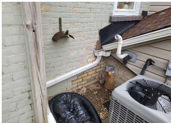
Photograph 35: View of the exposed buff brick on south elevation (AECOM, 2025)
