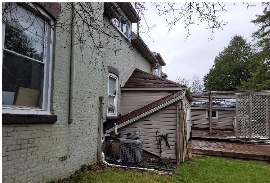
Photograph 43: View of the one-storey addition's west elevation (AECOM, 2025)
