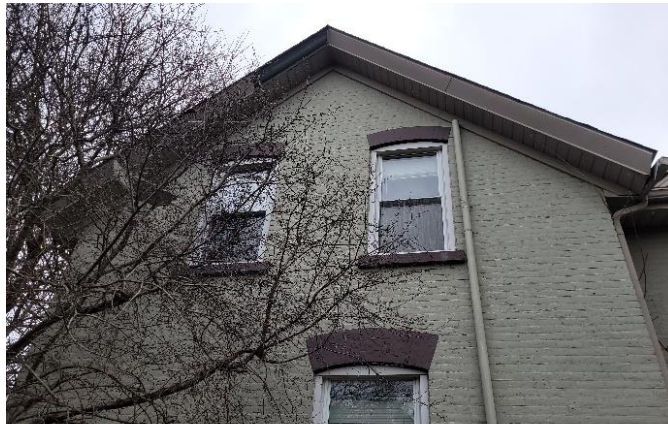
Photograph 38: View of the second storey windows on west wing of the south elevation (AECOM, 2025)
