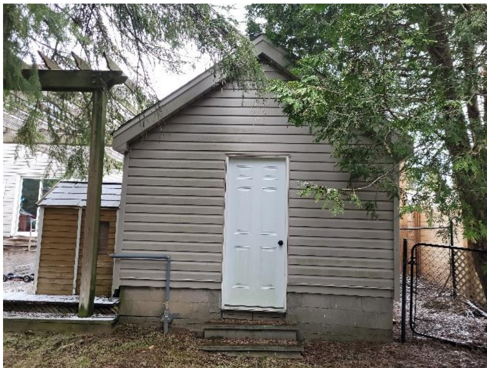
Photograph 44: View of the south elevation of the shed (AECOM, 2025)
