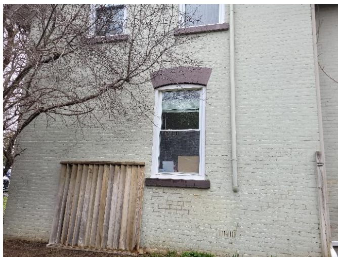
Photograph 37: View of the first storey window on west wing of the south elevation (AECOM, 2025)
