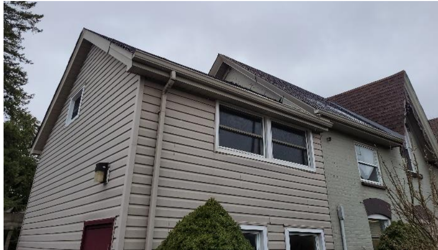
Photograph 26: View of the space between east addition and original farmhouse on east elevation (AECOM, 2025)
