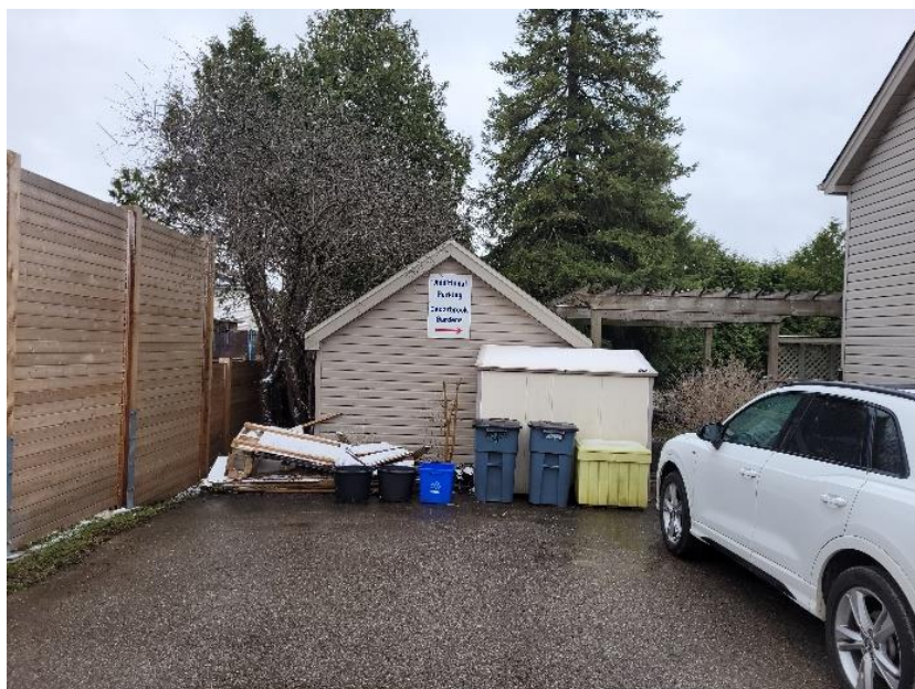
Photograph 46: View of the north elevation of the shed (AECOM, 2025)
