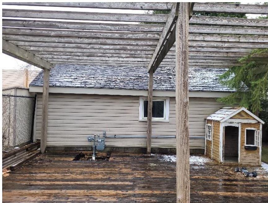
Photograph 47: View of the west elevation of the shed (AECOM, 2025)
