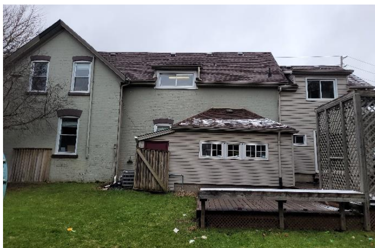
Photograph 29: View of the south elevation of the farmhouse (AECOM, 2025)
