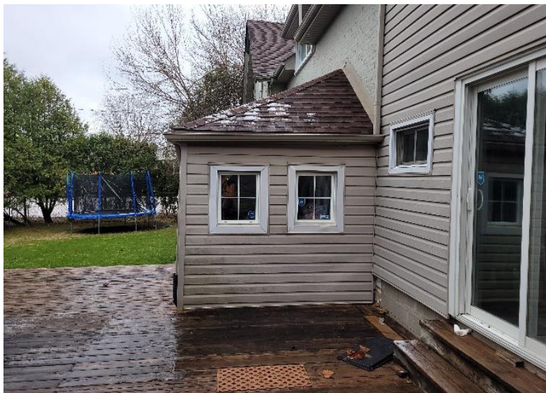
Photograph 28: View of the east elevation of the one-storey addition off south elevation (AECOM, 2025)
