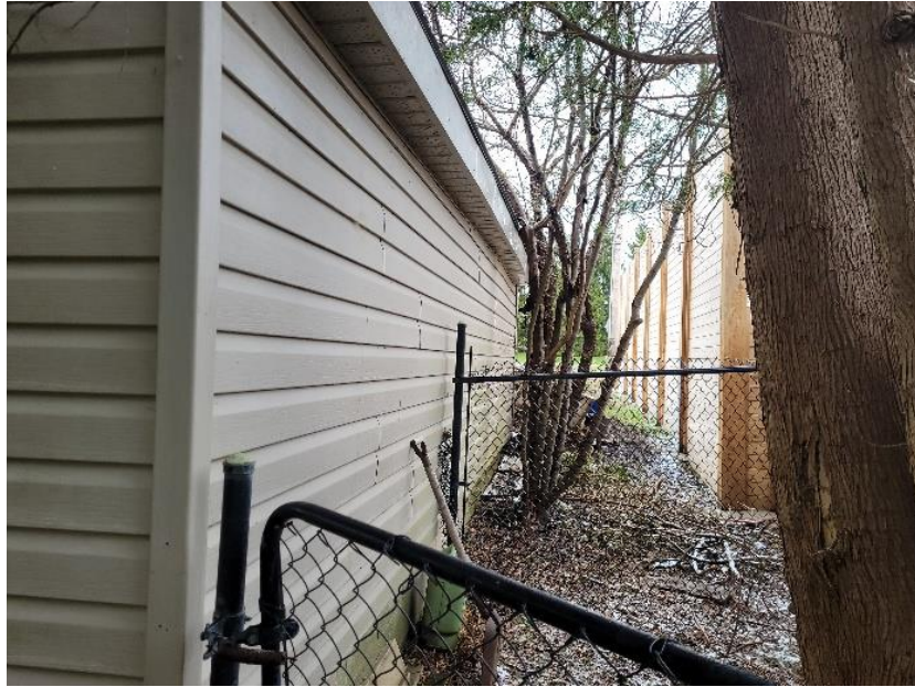
Photograph 45: View of the east elevation of the shed (AECOM, 2025)
