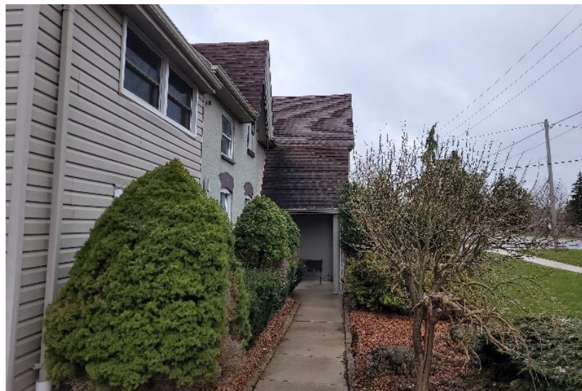
Photograph 27: View of the east elevation of the projecting wing and portico (AECOM, 2025)
