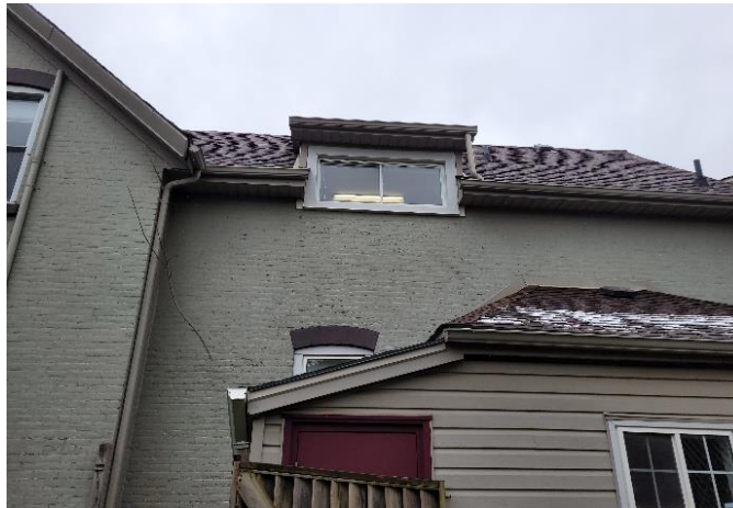
Photograph 36: View of the dormer and window in second storey of the south elevation (AECOM, 2025)
