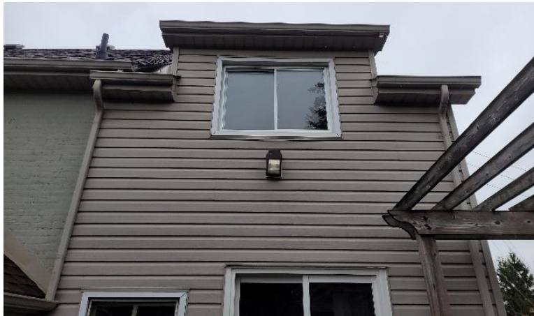
Photograph 32: View of the dormer on second storey of the east addition on south elevation (AECOM, 2025)
