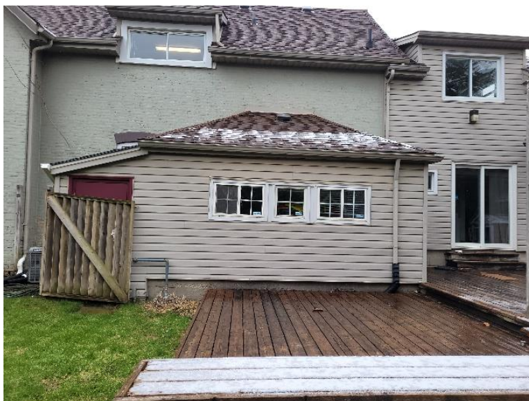
Photograph 33: View of the one-storey addition on south elevation (AECOM, 2025)
