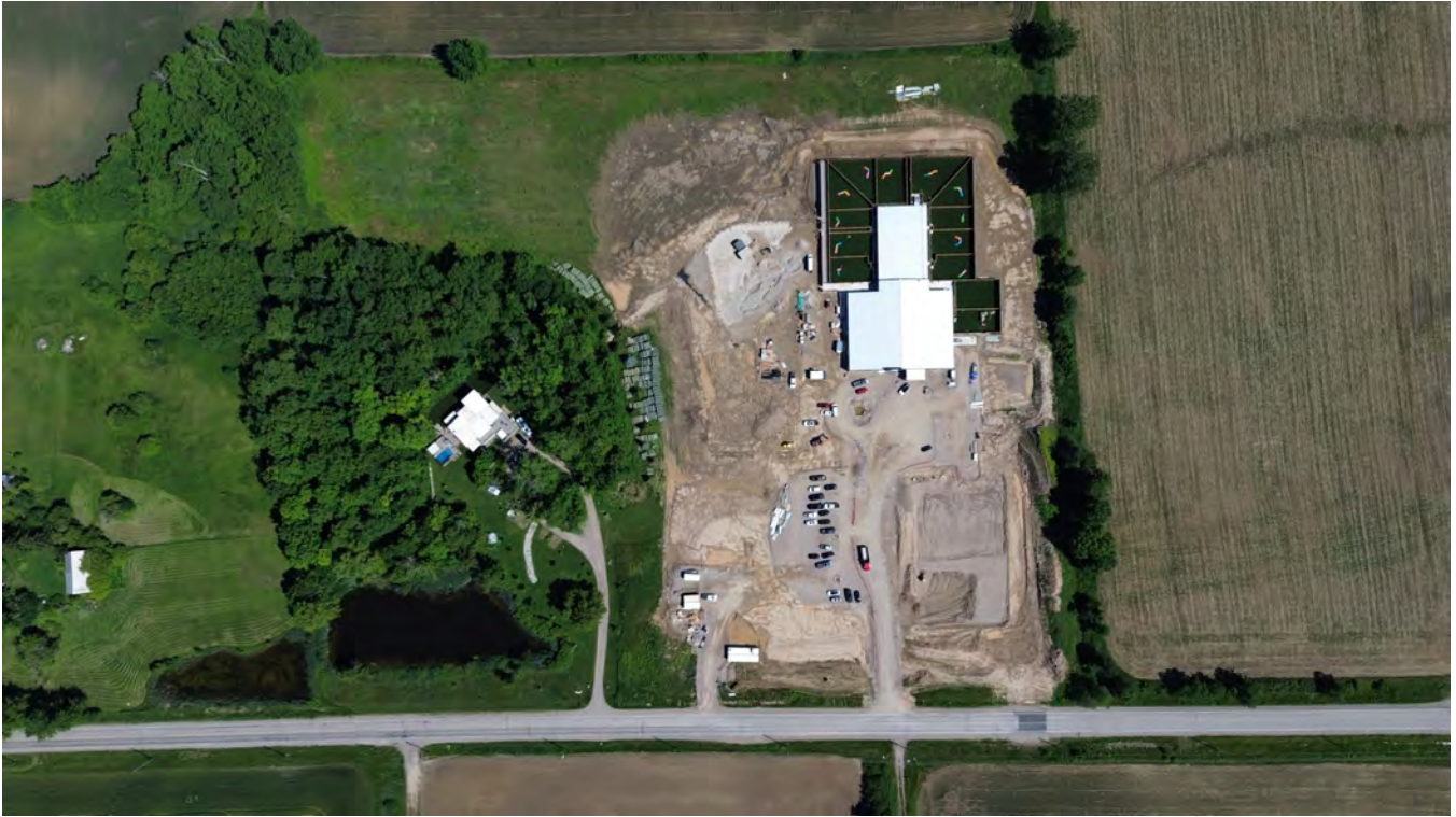
Site Photos: Top-down aerial view
