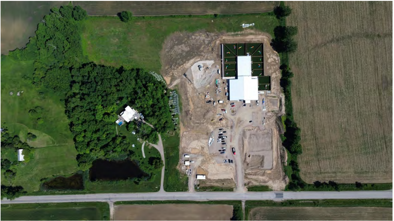
Site Photos: Top-down aerial view
