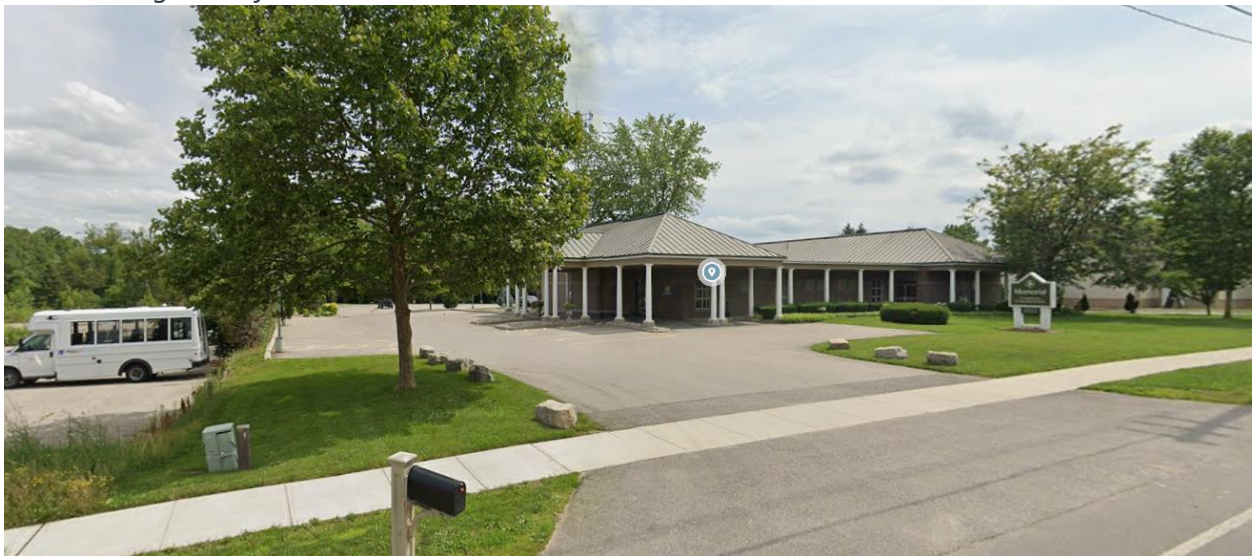
Figure 7 | Memorial Funeral Home Directly Abutting the Subject Lands View looking south from Fanshawe Park Rd E
