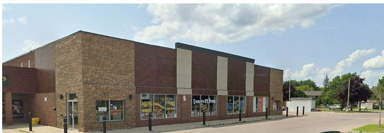
Figure 3 | Existing MN# 725 Buildings on Site
