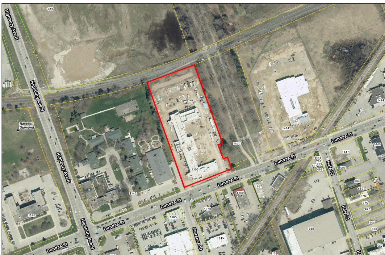
Figure 1- Aerial Photo of 1390 Dundas Street and surrounding lands.
