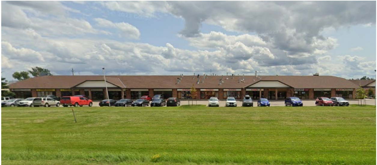
Figure 2 - Streetview of the subject lands (view looking south from Exeter Road)
