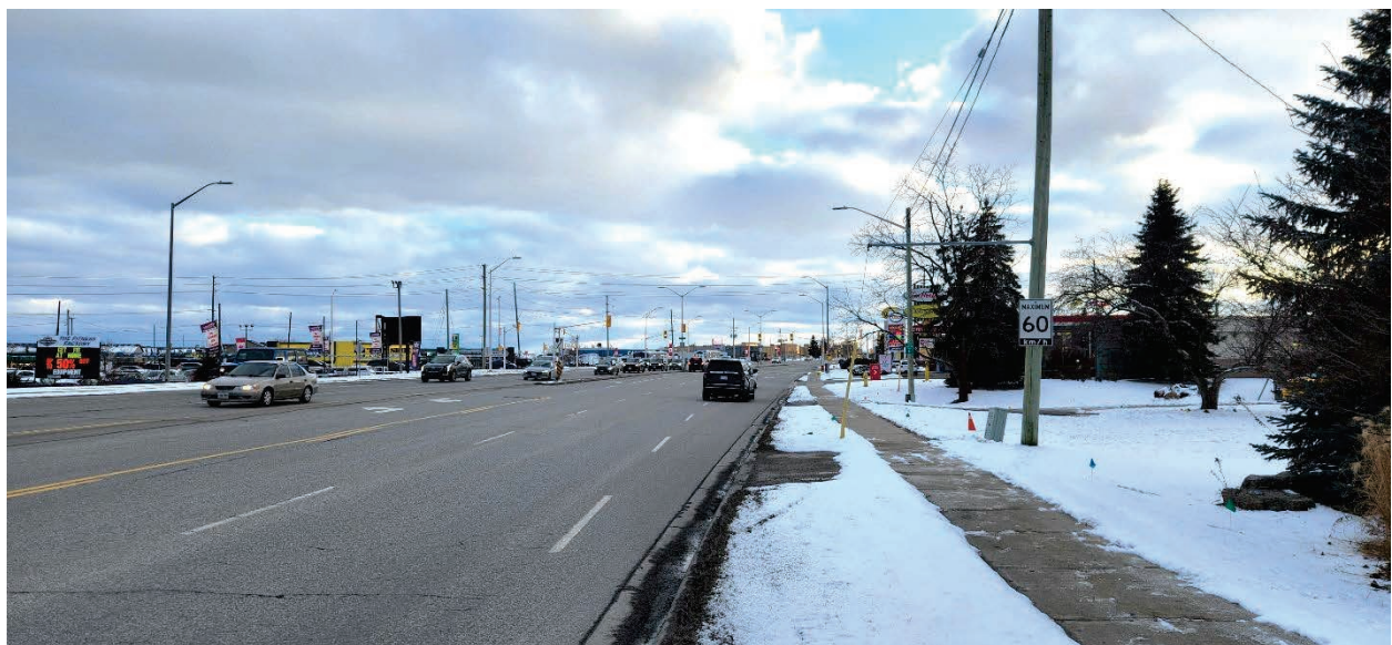
Figure 8: Wharnccliffe Road South, Looking South Towards Southdale Road East.
