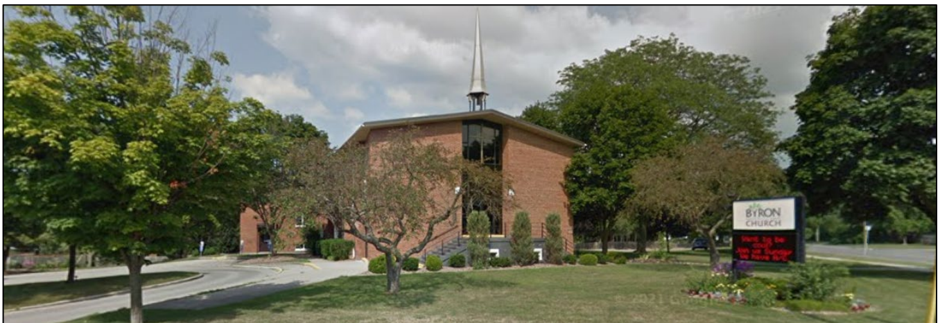
Photo 5. View of Byron United Church looking east from Boler Road.
