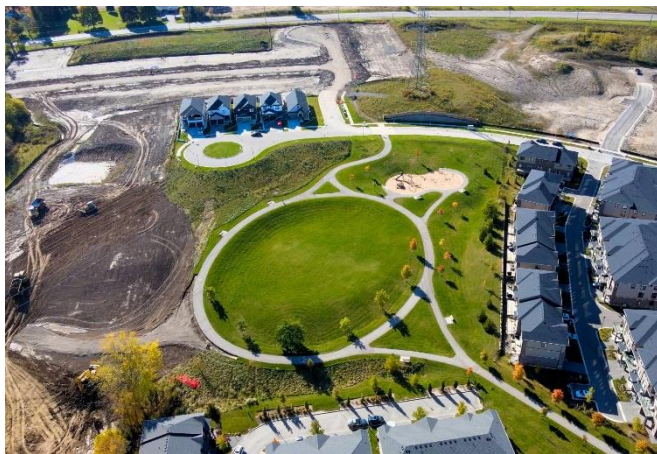
View towards Block 22 and Commissioners Rd. E from above.
