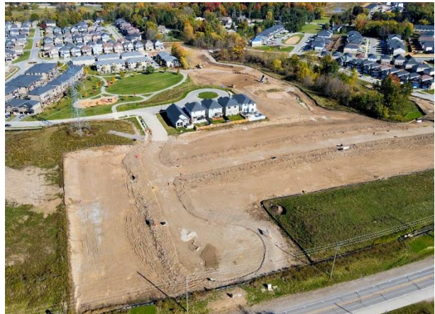
View to the north from Commissioners Road East (above)
