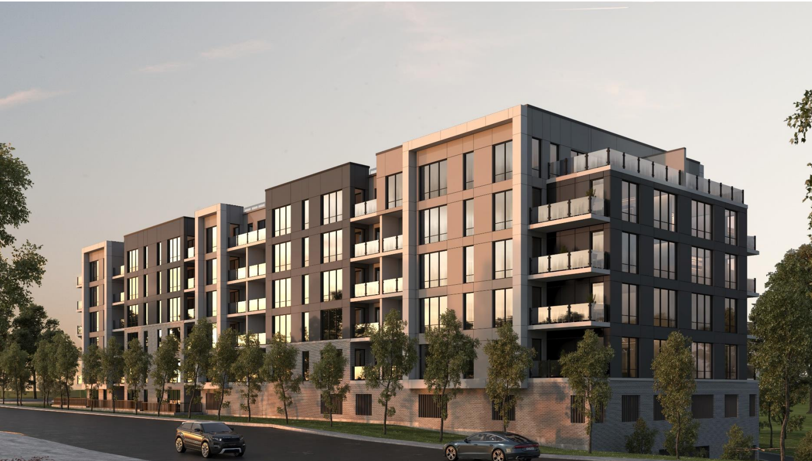
View of Block 22 from Commissioners Road East
