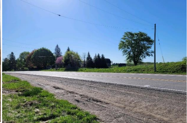
View to the southeast from Commissioners Road East
