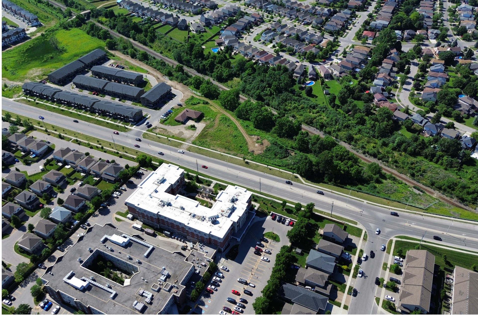
Figure 2. Aerial View of 801 Sarnia Road - NW Perspective
