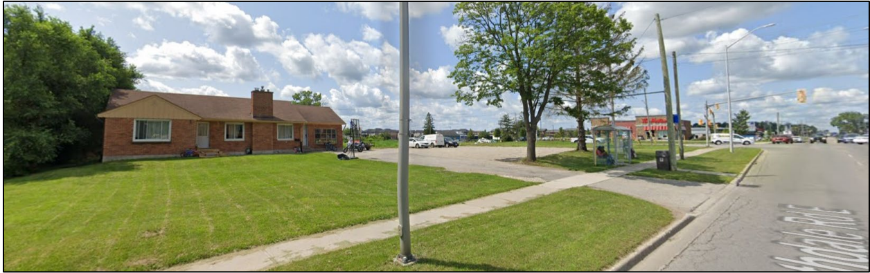
Figure 15 – Single detached dwellings on Petty Road (looking south)
