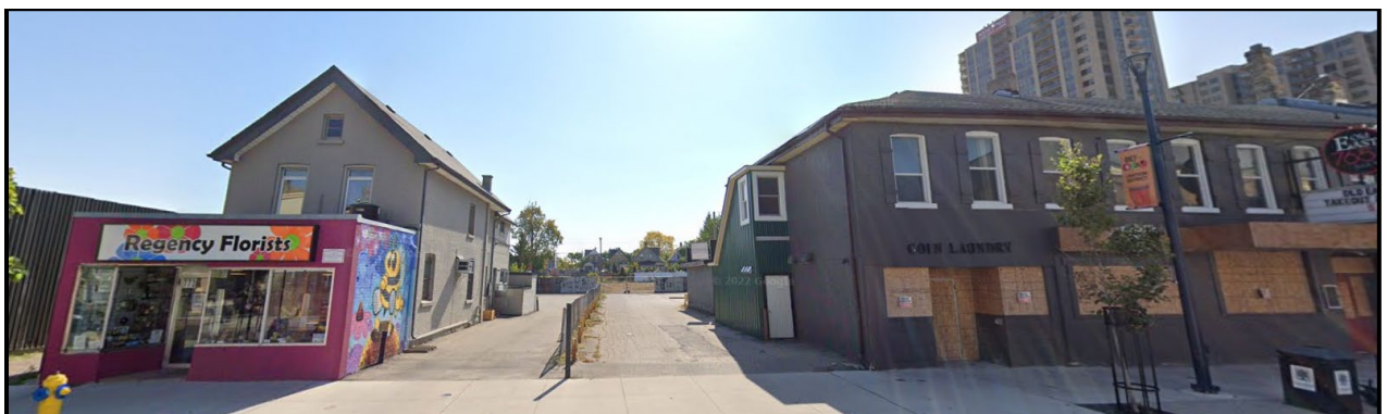
Figure 2 - Streetview of the subject lands (view looking south from Dundas Street)
