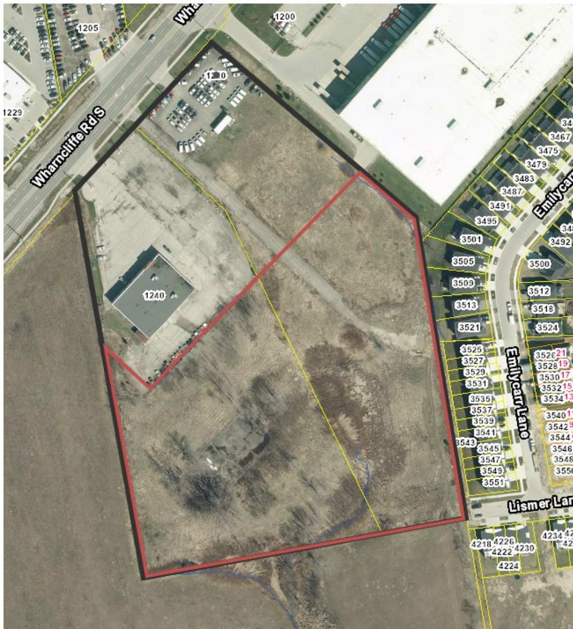
Figure 1- Aerial Image of 1210-1240 Wharncliffe Road S with subject parcel marked in red and larger parcel in black.
