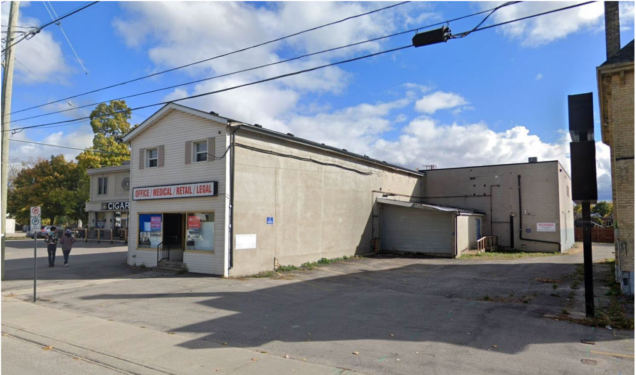
Figure 2 - Streetview of the Existing Vacant Commercial Building at 323 Horton Street East
