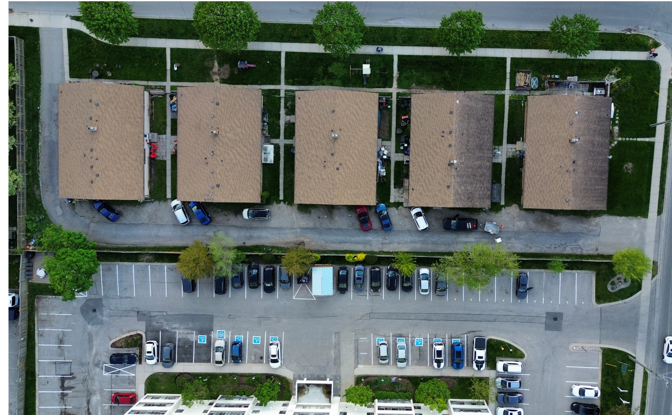
Note: Aerial view of existing conditions at 145 Base Line Road West.
