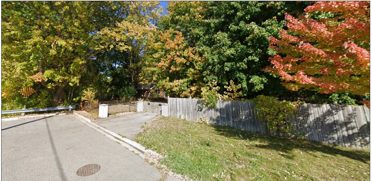
Figure 2 - Streetview of 32 Chesterfield Avenue (view looking northeast)
