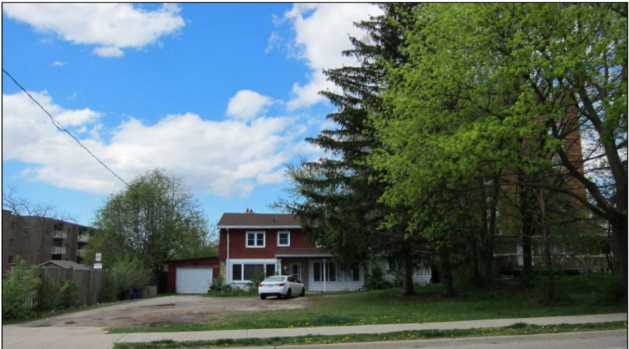
Figure 3 - Streetview of 82 Base Line Road West (view looking north)
