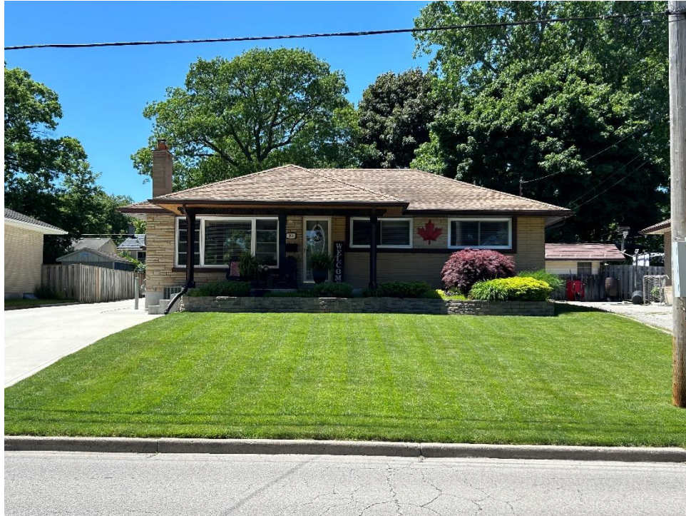
Figure 7 – Example of Single-Detached Dwelling on Griffith Street
