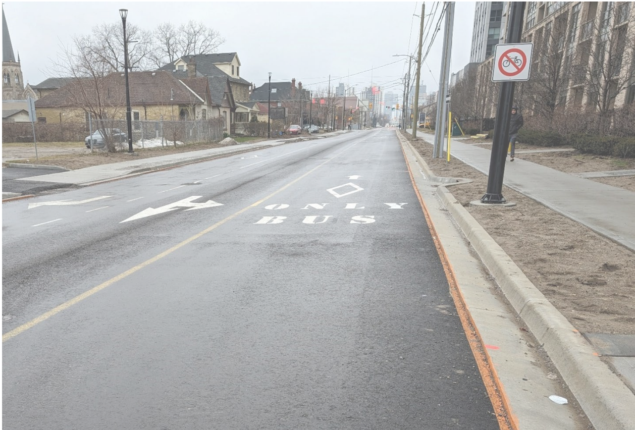
West Leg of Hewitt Street at King Street
