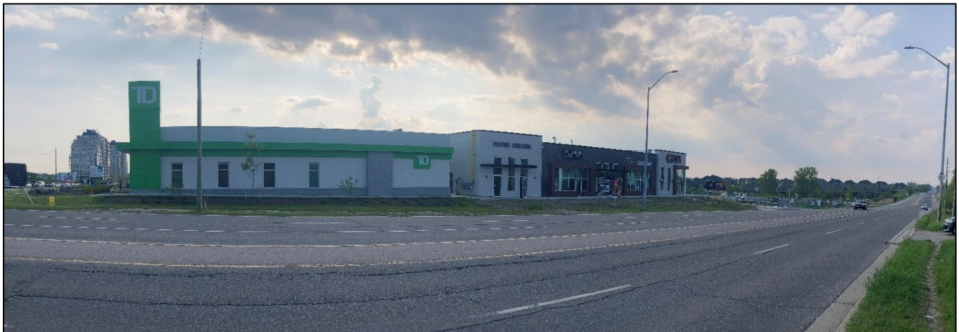
Figure 4. Commercial development on Richmond Street to the west of the subject site.
