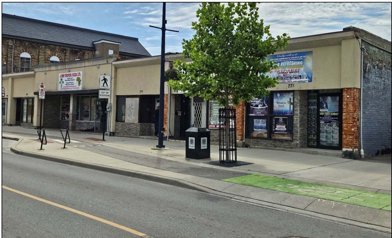
Image 4 – Dundas Street right-of-way
