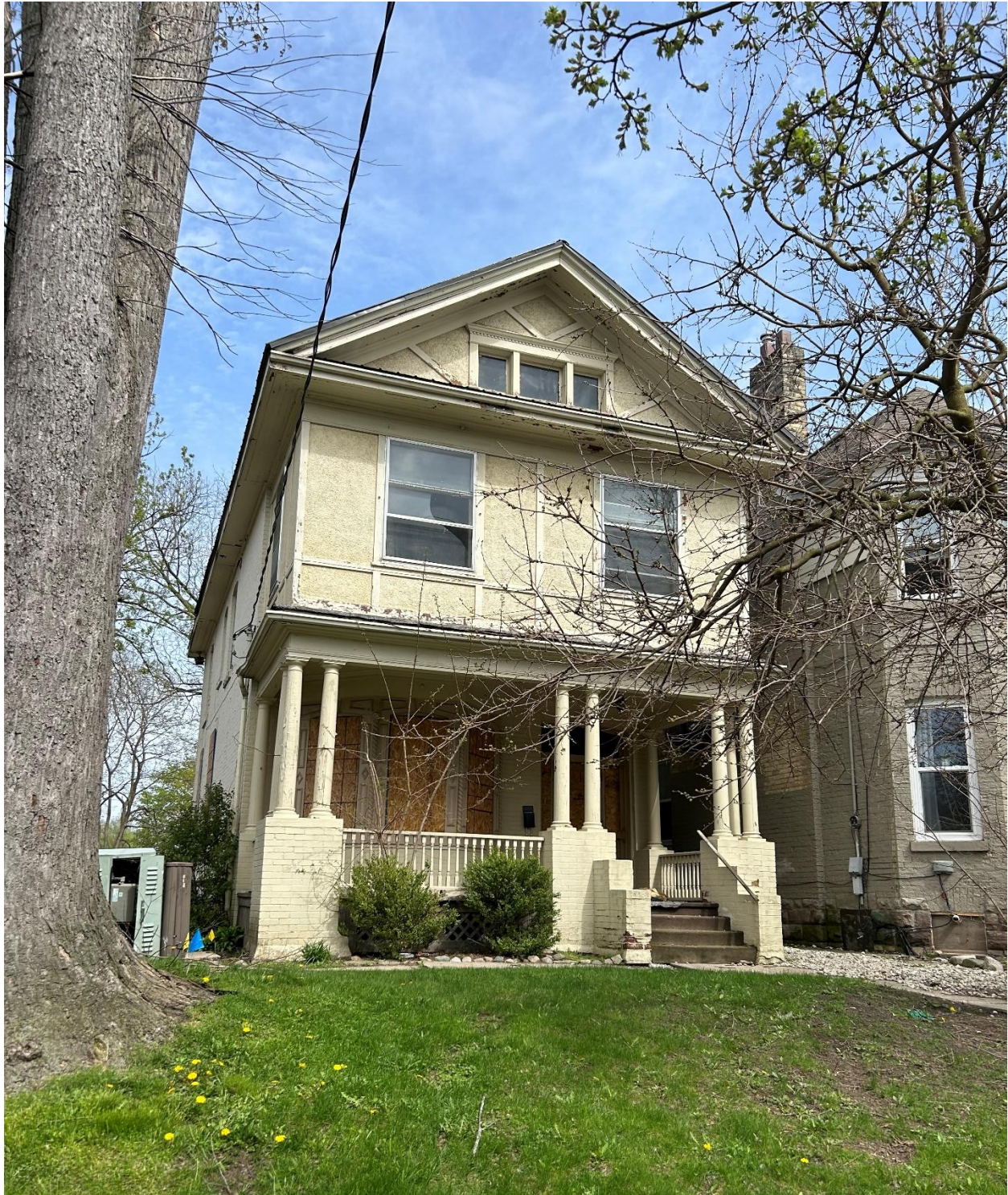
Figure 3: Street view of 572 Colborne Street
