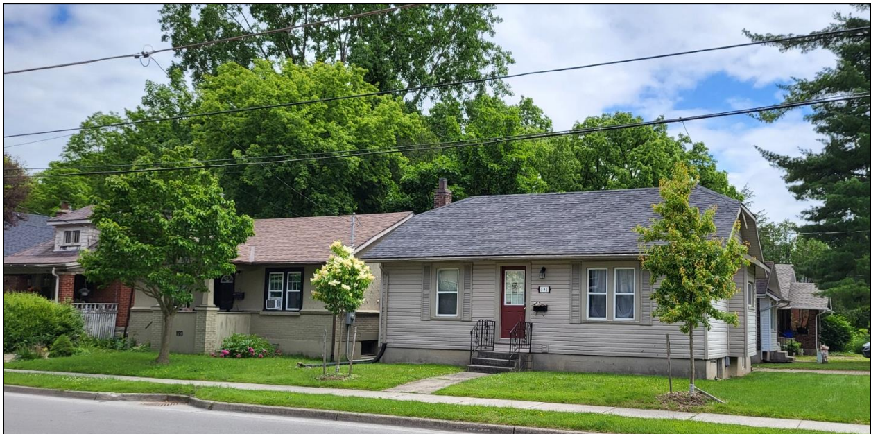
Figure 15: Single-detached dwellings south of the subject lands on Huron Street
