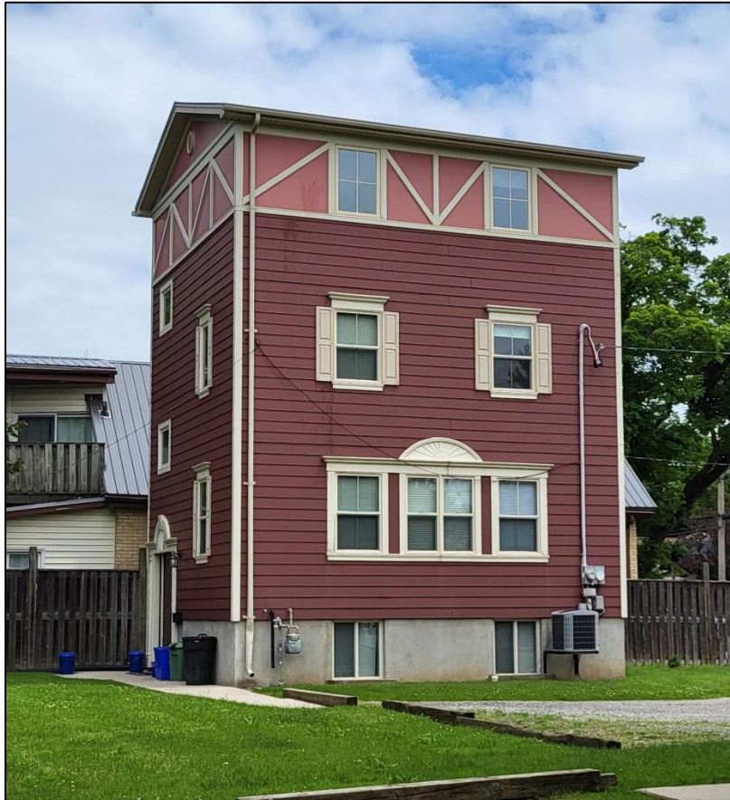
Figure 6: Existing 3-storey residential dwelling at 188 Huron Street
