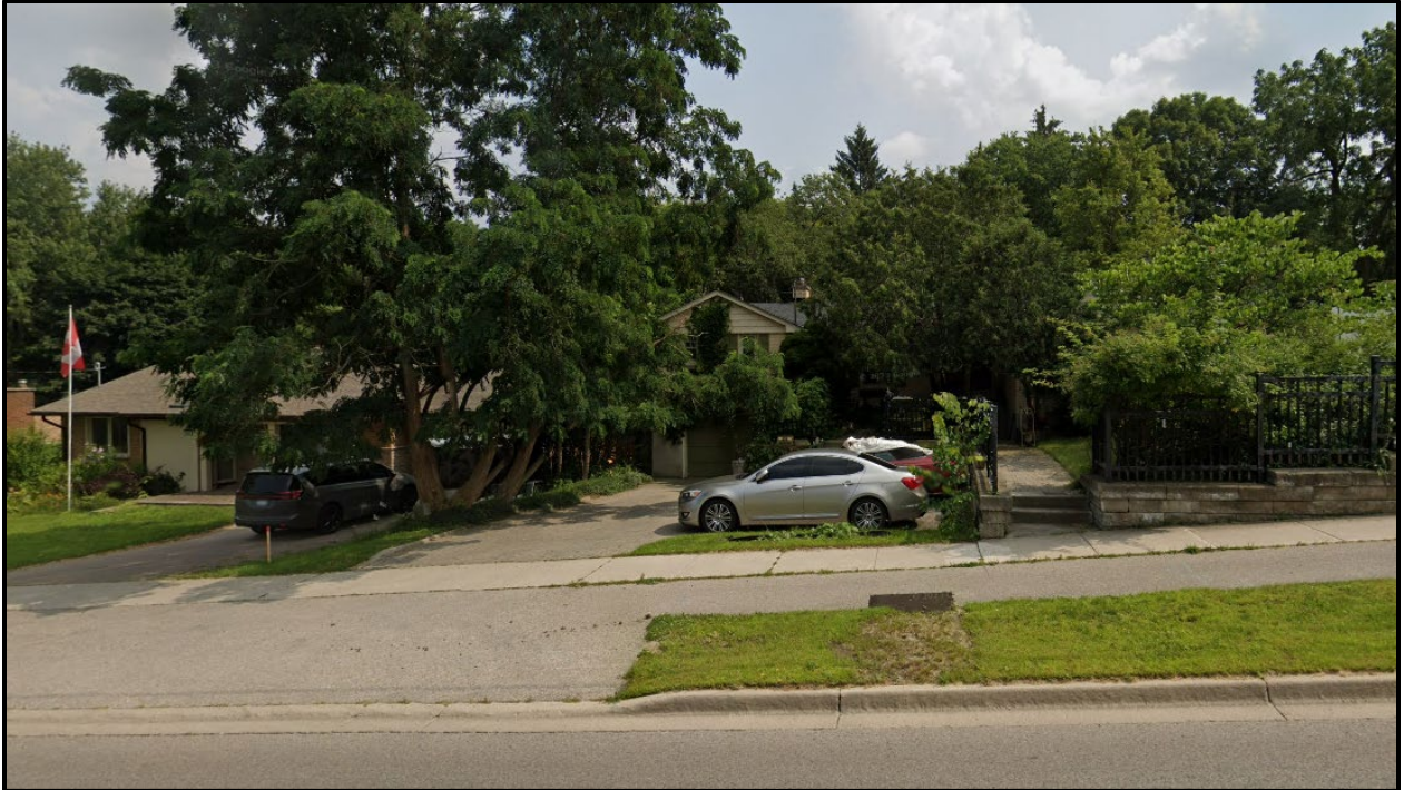
Figure 2 - Streetview of 934 Oxford Street West (view looking south)
