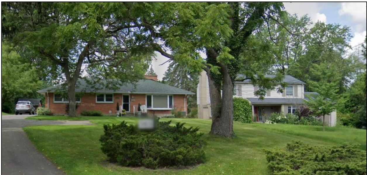
Figure 5 – 'Ranch' (left) and 'Typical 2-storey' (right) suburban homes along Upper Queen Street
