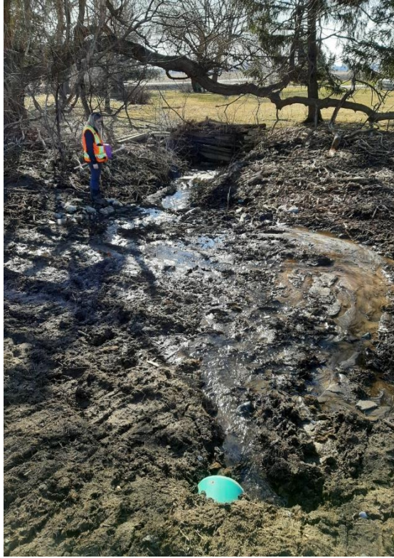
Photograph No. 3 – Culvert in Community 3 on March 17, 2022
