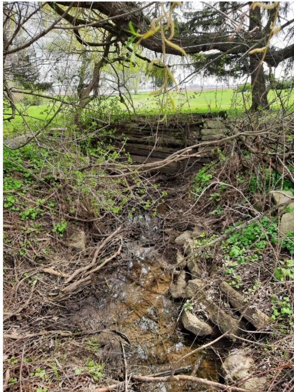
Photograph No. 6 – Culvert in Community 3 (April 23, 2021).
