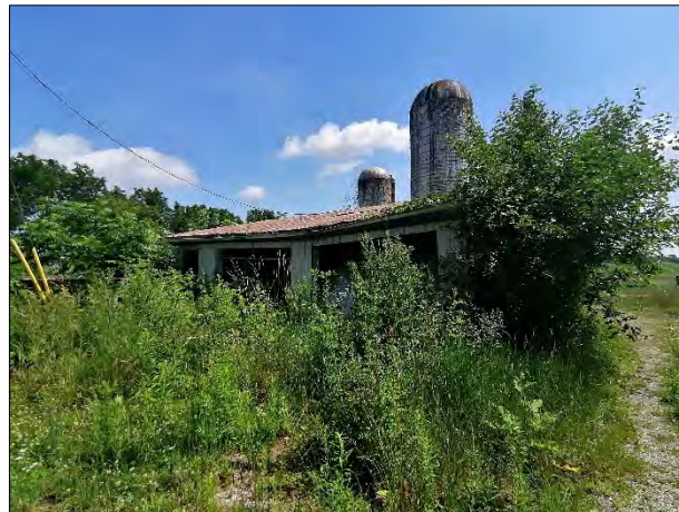
Figure 25: View of outbuilding 2 looking east (MHBC, 2021)
