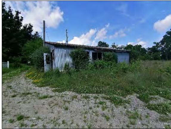
Figure 24: View of outbuilding 1 looking east (MHBC, 2021)
