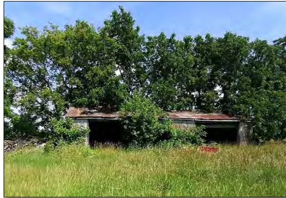
Figure 26: View of outbuilding 3 looking north (MHBC, 2021)
