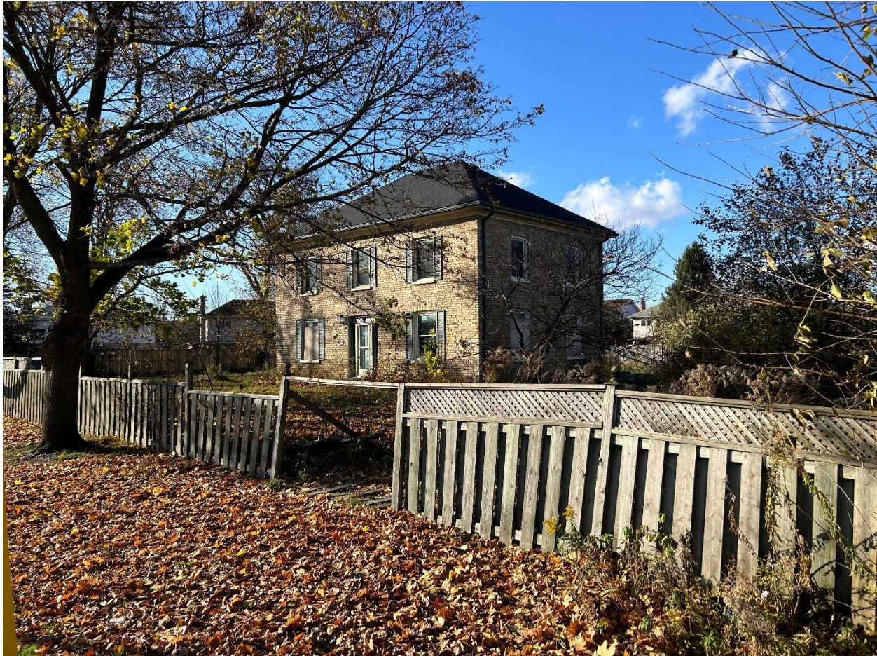
Figure 2: Existing Building on Subject Lands
