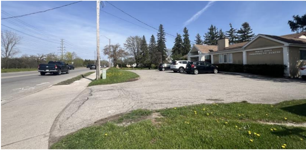
Figure 2 – Access asphalt driveway and parking area
