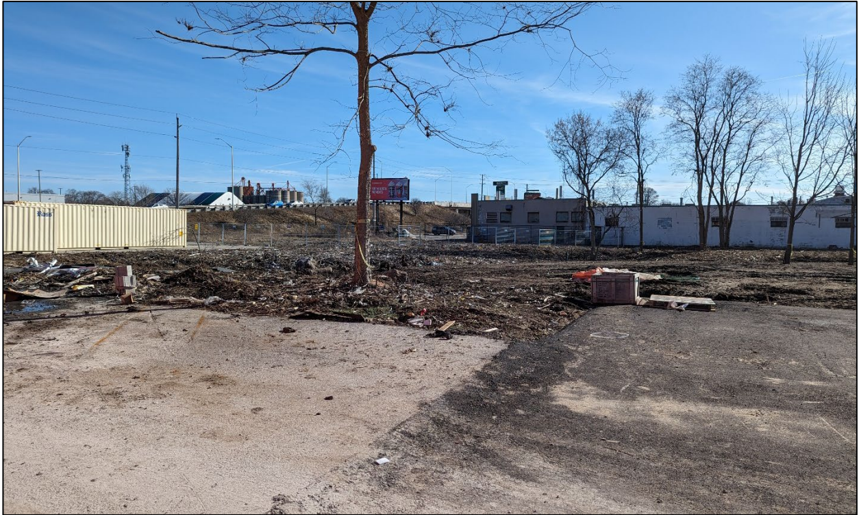
Figure 4 – Subject Lands, looking southeast
