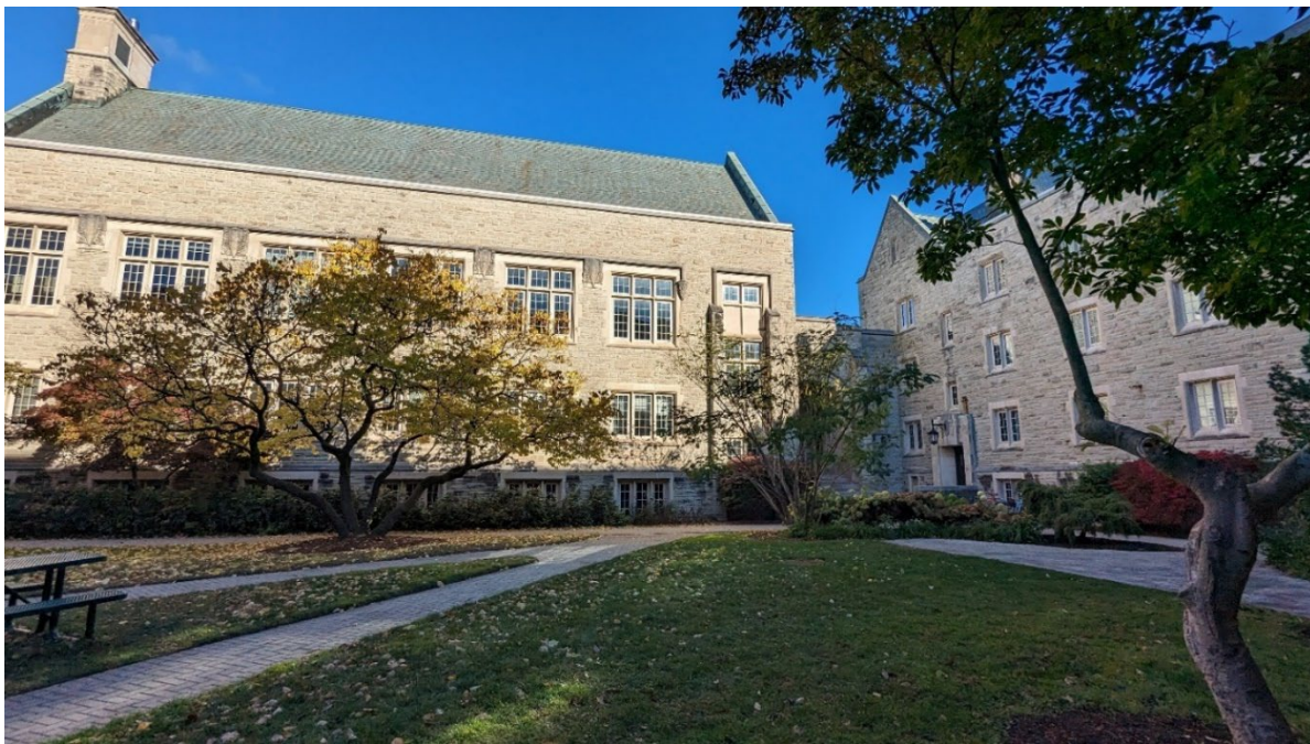
Photos 44-46: (above) View of front (north) elevation from the internal courtyard looking towards the front entryway; (below) View of internal courtyard looking towards front entryway (MHBC, 2023).
