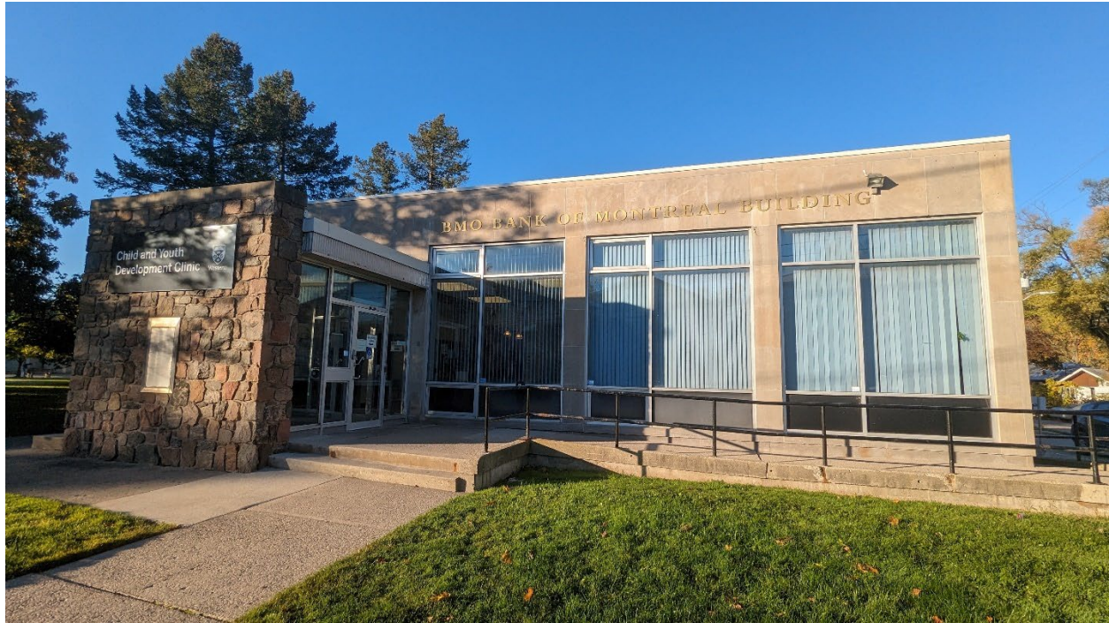
Photo 7: View of the BMO Bank of Montreal Building located at 1163 Richmond Street which is part of the Project Site (MHBC, 2023)
