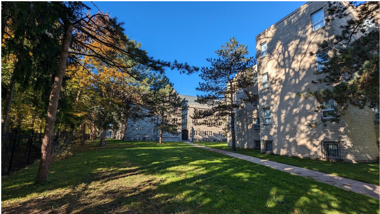
Photos 36 & 37: (above) View of north (front) elevation of Medway Hall looking southwards from north side of University Drive; (below) View of east elevation of Medway Hall and rear elevation of Alumni House looking westwards (MHBC, 2023).
