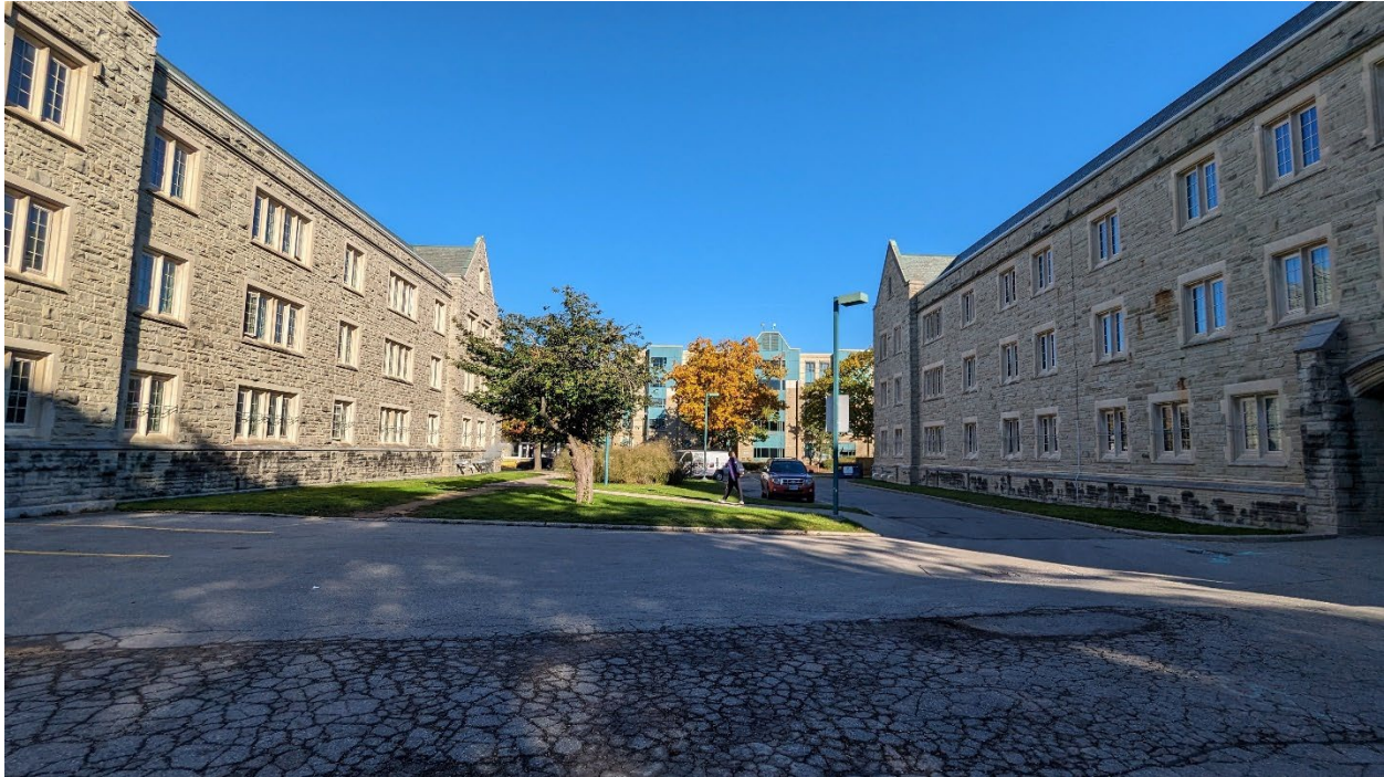
Photo 51: View of western elevation of Medway Hall (MHBC, 2023).
