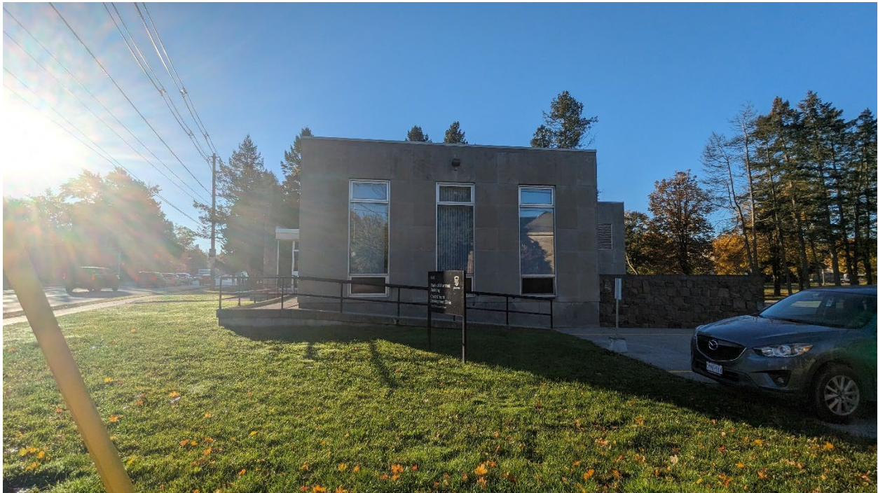
Photos 57 & 58: (above) Perspective view of east (front) elevation and north elevation of the building looking south-west; (below) View of north elevation of building looking southwards (MHBC, 2023).
