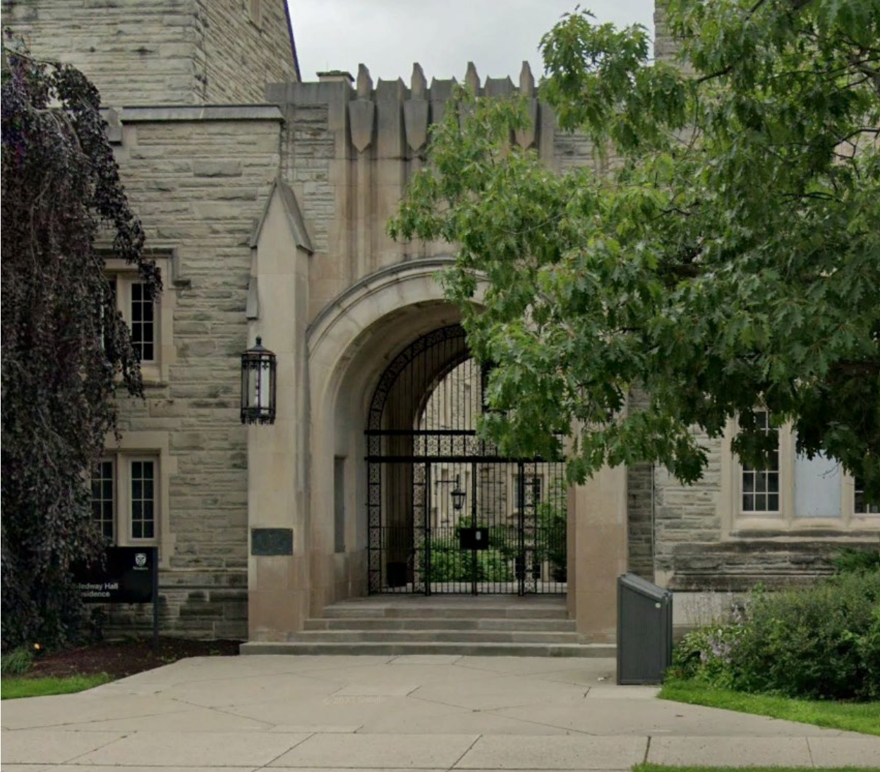
Photo 33: Main entryway of Medway Hall (MHBC, 2023).
