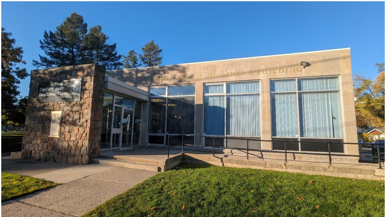
Photos 55 & 56: (above) View of east (front) elevation of the building looking north-west; (below) View of east elevation of building looking westwards and towards vestibule entrance and feature stone wall (MHBC, 2023).
