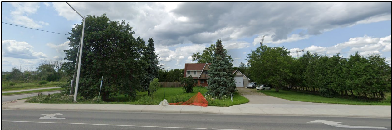
Figure 2 - Streetview of 1467 Wharncliffe Road South (view looking northwest from Wharncliffe Road S)
