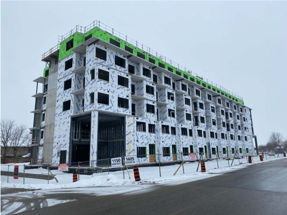
Photo 5 – View of six-storey apartment building, west of subject lands, across Stackhouse
