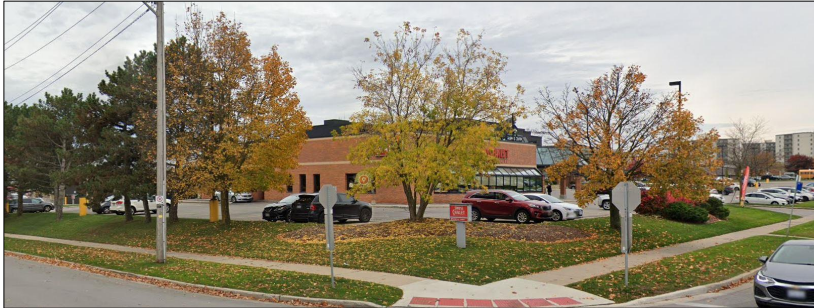
Figure 2. Subject site and proposed Development Area, looking southwest from Beaverbrook and Horizon intersection (Google Streetview).
