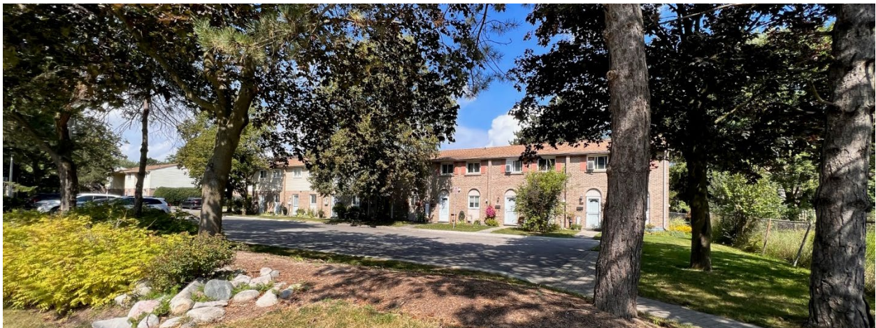
Figure 5 – Street View of Townhouses West of the Subject Lands
