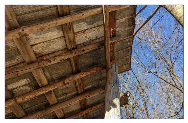
Photo 47: Detailed view of supports and metal sheeting
