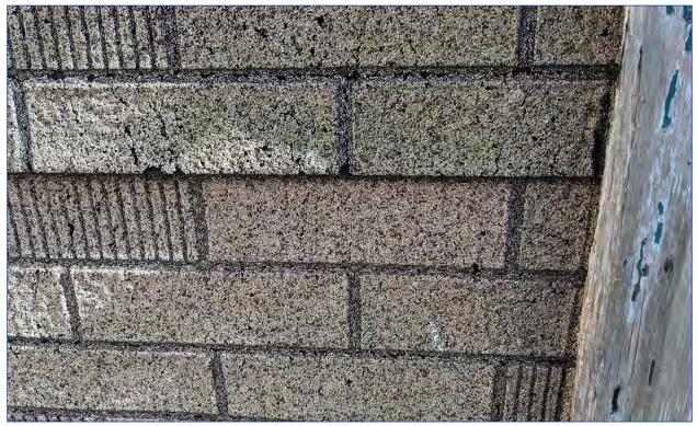
Photo 15: Detailed view of the insulbrick type cladding on the enclosed front porch area on the south elevation
