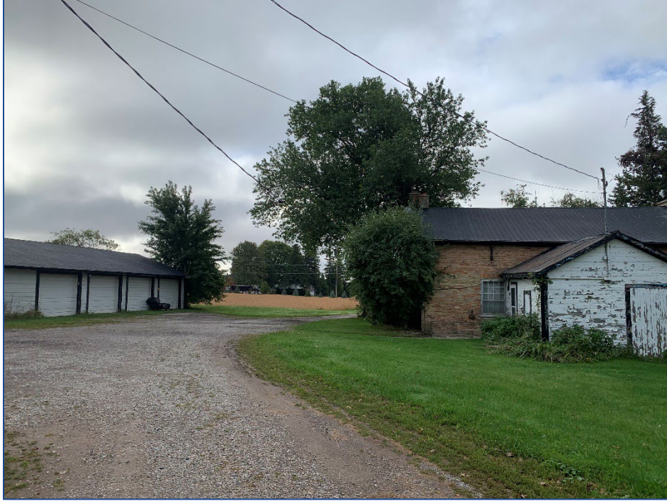
Photo 3. Anthropogenic area (AN) in the southeastern portion of the Subject Property September 28, 2022).
