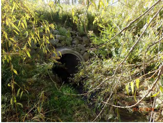
Photo 7. Upstream Culvert under Sunningdale Road (October 2018).
