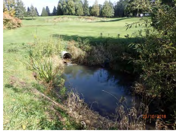
Photo 10. Axford drain culvert from Pond facing north (June 2018).
