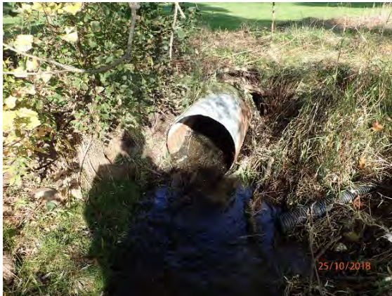
Photo 8. Culvert along Axford Drain north of Sunningdale Road (October 2018).
