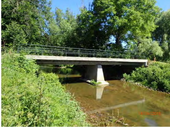
Photo 18. Cart Bridge across Medway Creek looking north from 6 Thompson.
