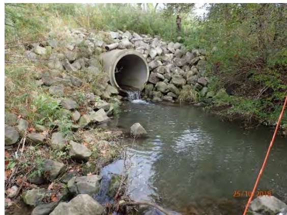
Photo 6. Culvert at Downstream side of Sunningdale Road (October 2018).
