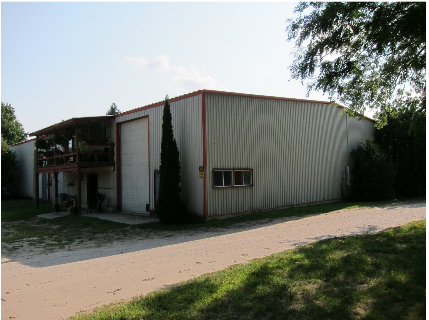
Figure 6. 1084 Crumlin Sideroad – large barn
