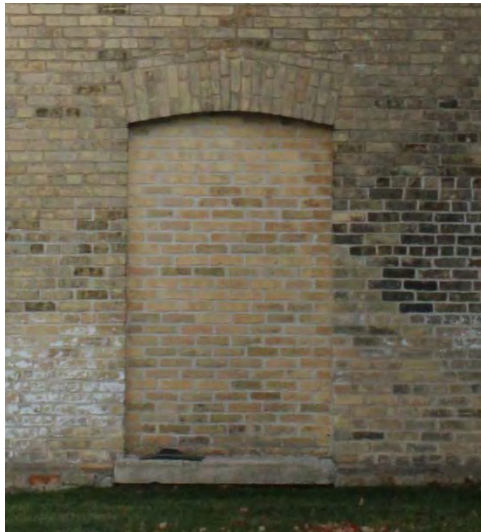
Figure No. 124: Door W-D3 – Hayloft Doors (Photo No. 25.6)
