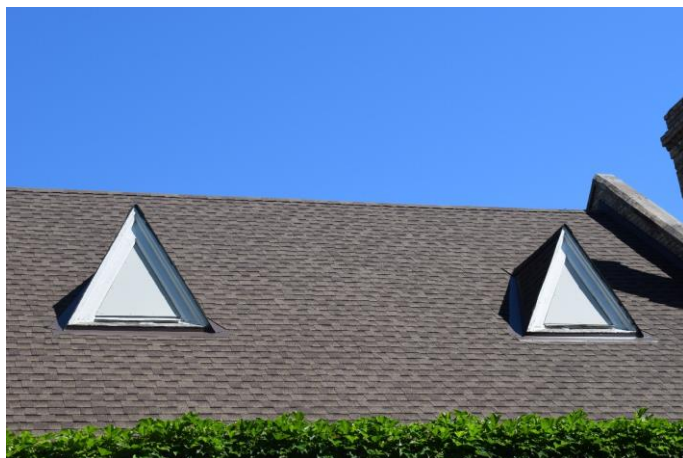
Photo 22: Chapel of Hope close-up of north elevation dormers
