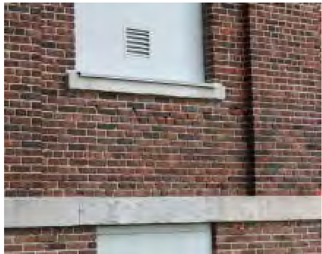
Figure No. 326: West Elevation (Centre) Stone Band Detail (Photo No. 21.3)
