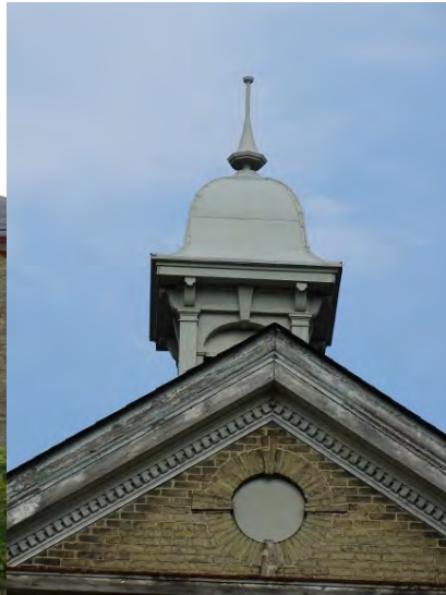
Figure No. 163: East Wing – North Elevation – Detail (Photo No. 78.2)
