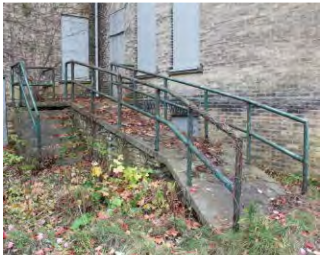
Figure No. 277: Central Pavilion and Corridors (Photo No. 109.1)
