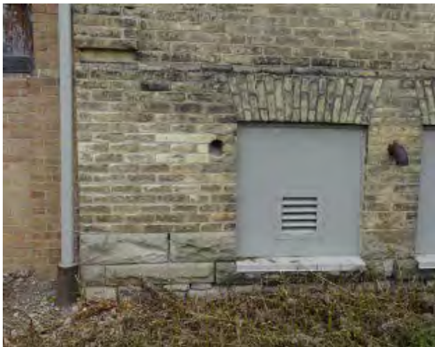
Figure No. 222: West Wing – South Elevation (Photo No. 98.1)
