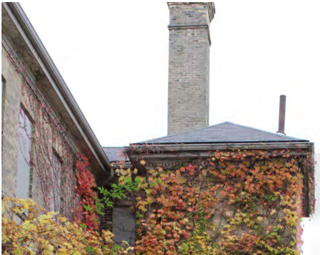
Figure No. 134: East Wing – Stair Tower – East Elevation (Photo No. 30.0)
