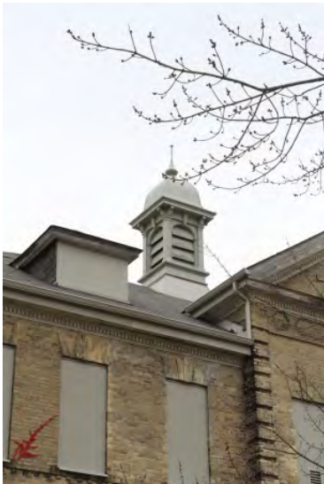
Figure No. 164: West Wing – South Elevation (Photo No. 79.3)
