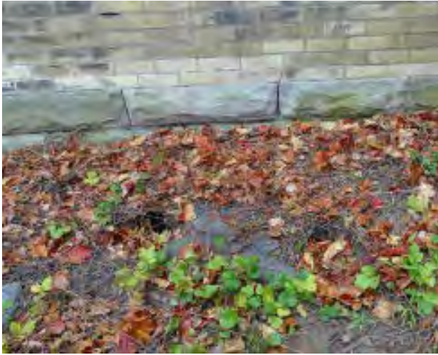
Figure No. 208: Central Pavilion and Corridors – South Corridor – West Elevation (Photo No. 92.1)
