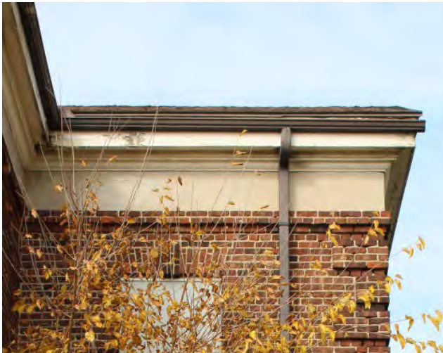
Figure No. 305: Rear East Wing East Pediment South Return (Photo No. 11.5)
