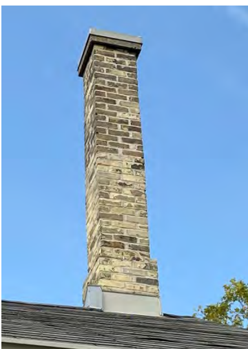
Figure No. 90: Chimney (Photo No. 14.0)
