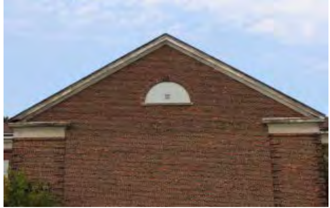
Figure No. 298: South Elevation, South Gable (Photo No. 11.0)
