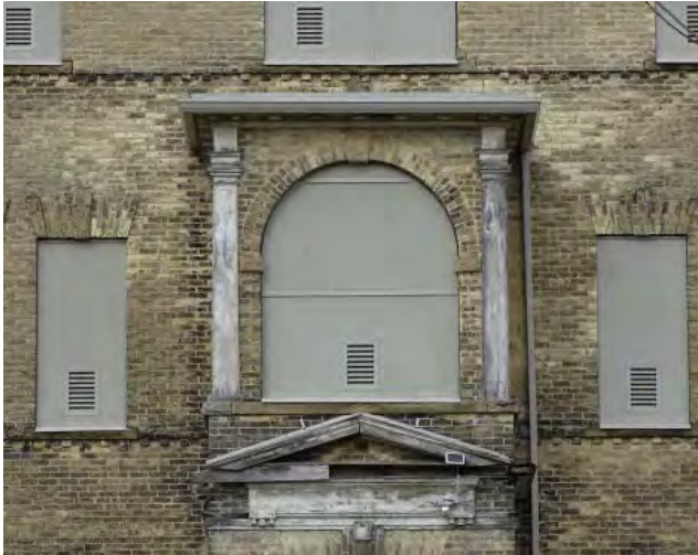
Figure No. 182: Central Administration Block – Entrance – South Elevation (Photo No. 80.0)
