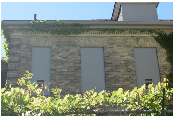
Photo 41: Infirmary close-up of dentilated cornice on rear elevation of east wing
