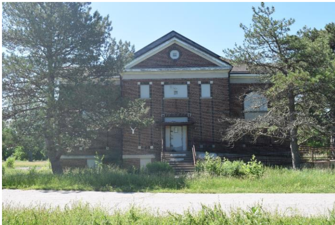
Photo 53: Recreation Hall north (main) elevation looking south
