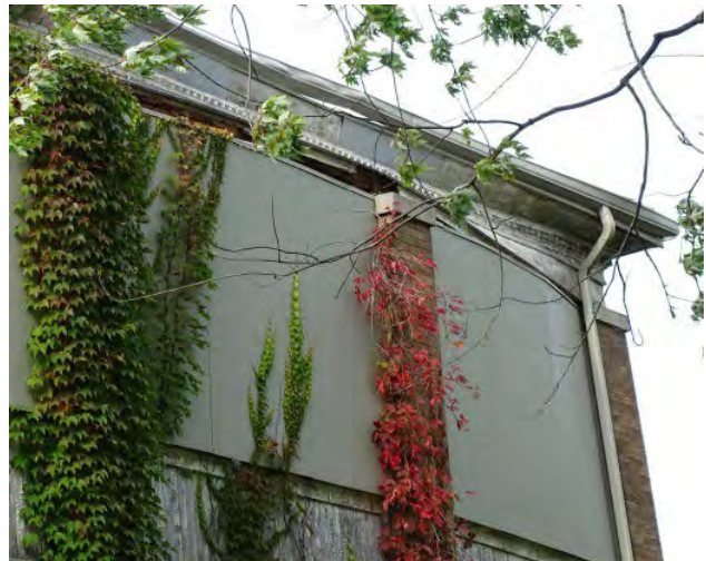
Figure No. 135: East Wing – Porches – East Elevation Detail (Photo No. 101.2)
