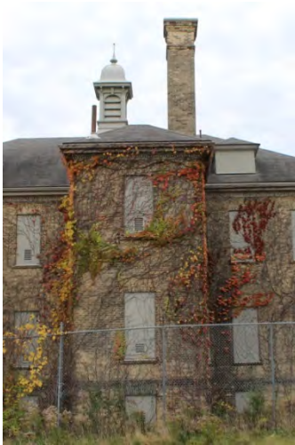
Figure No. 174: East Wing – Stair Tower Chimney – North Elevation (Photo No. 74.0)
