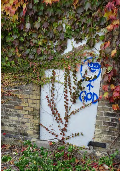
Figure No. 67: Door E-D2 (Photo No. 33.2)
