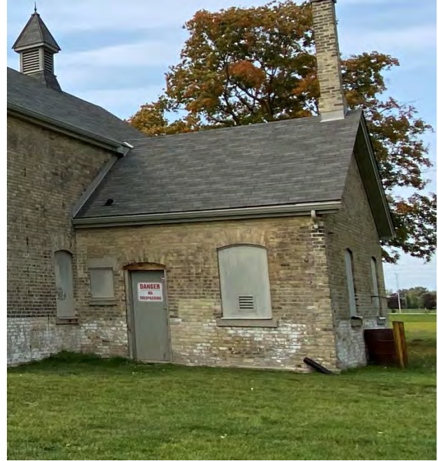
Figure No. 103: South Elevation (Photo No. 18.0)
