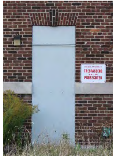
Figure No. 340: Door E-D1 (Photo No. 27.1)
