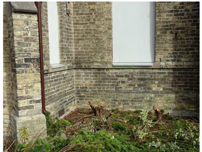
Figure No. 55: West Elevation – West/Main Entrance Visible Stone Foundation (Photo No. 31.0)
