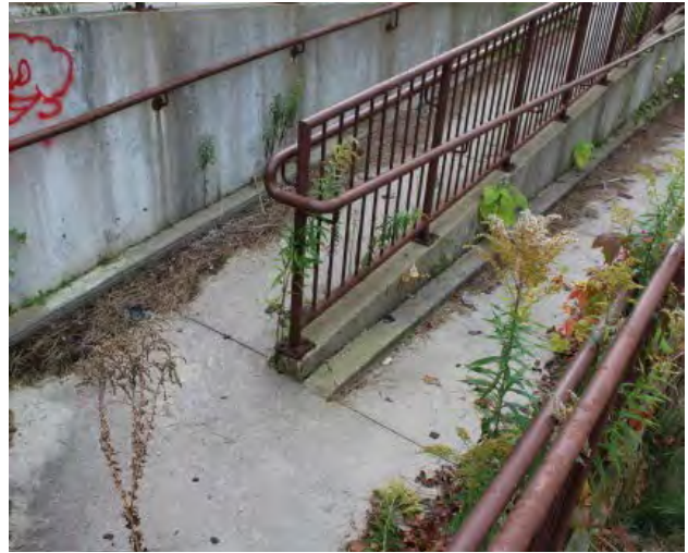
Figure No. 347: North Elevation, Ramp Detail (Photo No. 28.4)
