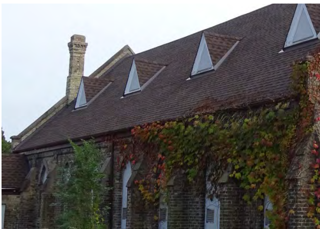
Figure No. 14: North Elevation – Nave Fascia (Photo No. 9.3)
