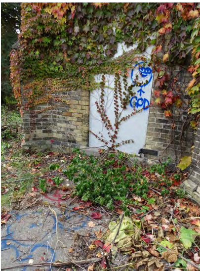
Figure No. 42: East Elevation – South Entrance Wing (Photo No. 21.12)
