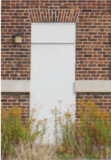
Figure No. 343: Door W-D2 (Photo No. 27.4)
