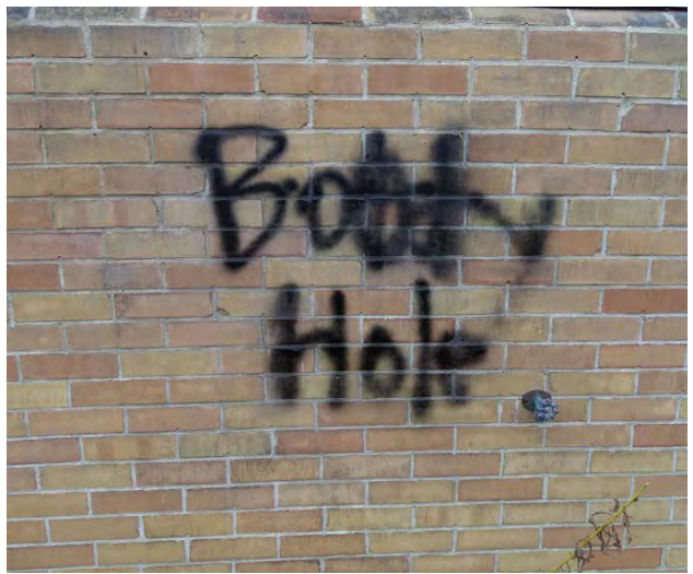
Figure No. 205: West Wing – West Porches – West Elevation (Photo No. 104.5)
