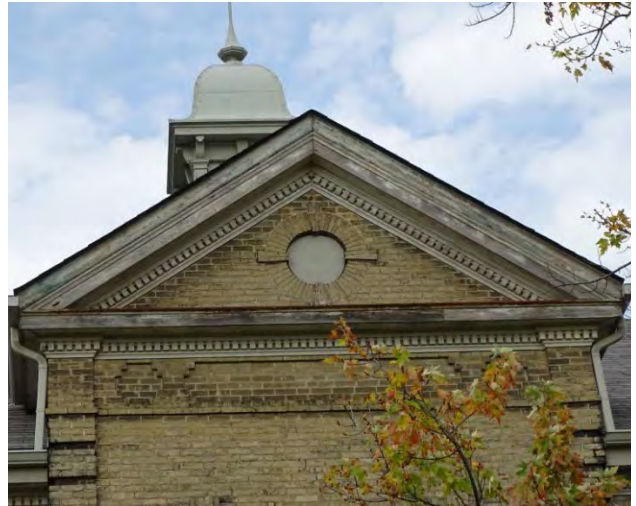
Figure No. 151: West Wing – East Elevation Detail (Photo No. 52.4)
