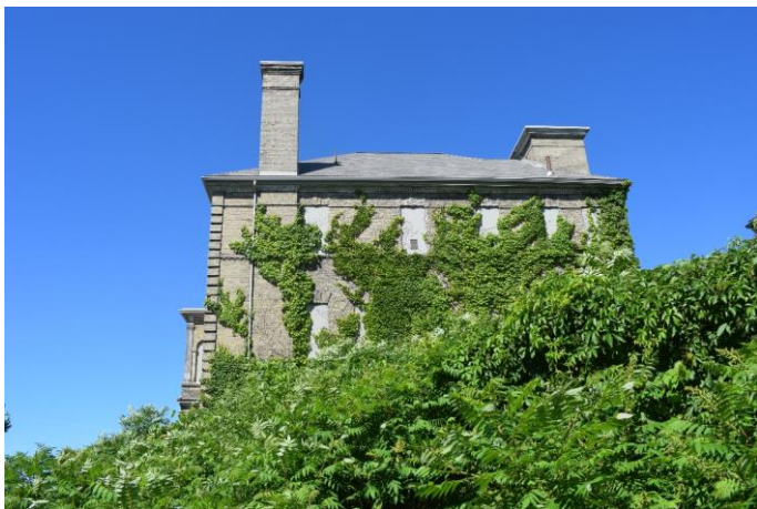
Photo 29: East elevation of Administration Block looking west
