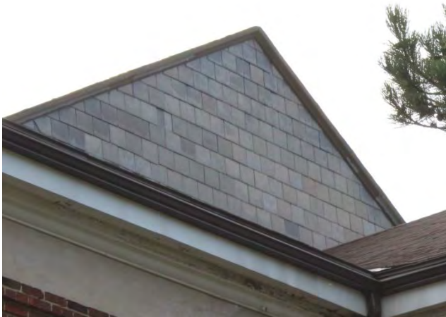
Figure No. 283: North Gable Slate Detail (Photo No. 5.1)
