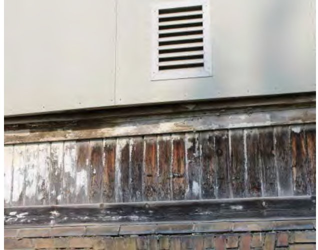
Figure No. 149: East Wing – Porches – South Elevation Detail (Photo No. 102.4)
