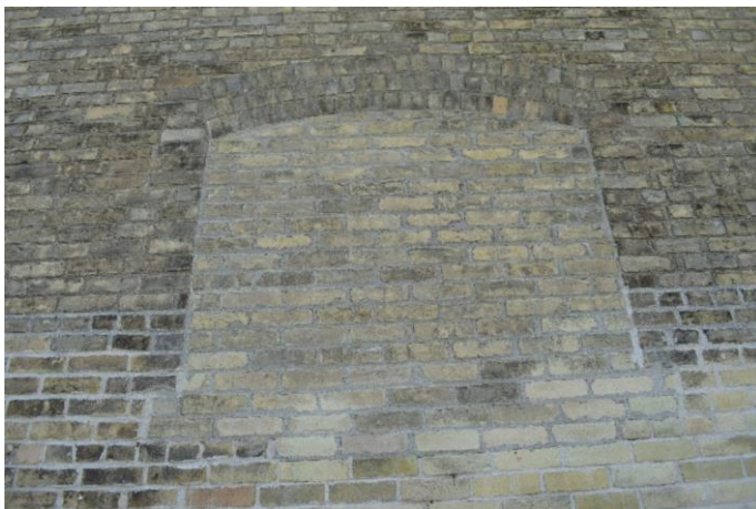
Photo 17: Horse Stable close-up of infill window
