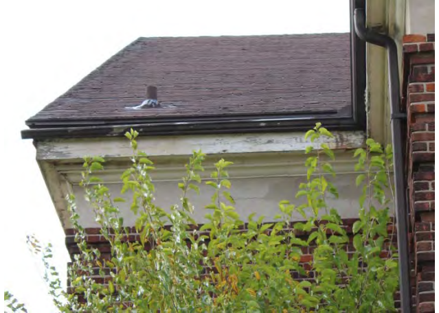
Figure No. 284: East Elevation Main Roof South of Rear East Wing (Photo No. 6.3)
