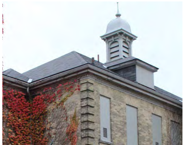
Figure No. 137: West Wing – East Elevation Detail (Photo No. 34.0)
