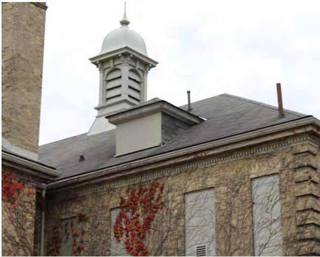
Figure No. 178: East Wing – North Elevation – North West Dormer (Photo No. 76.1)
