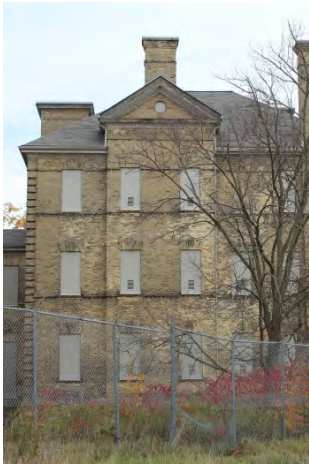
Figure No. 166: Central Administration Block – West Chimney – West Elevation (Photo No. 70.0)
