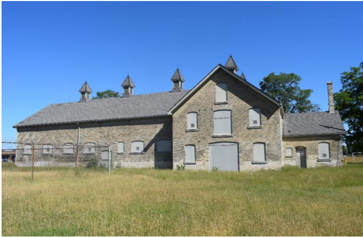
Photo 1: Horse Stable south elevation looking northwest
