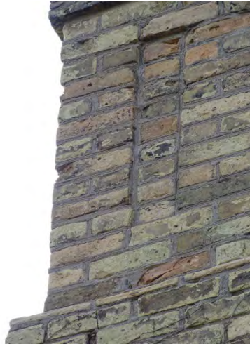
Figure No. 27: East Gable – North Chimney – Detail (Photo No. 17.5)
