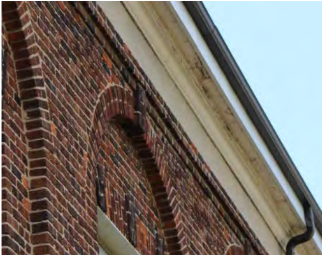
Figure No. 293: East Elevation Main Roof (Centre) Detail (Photo No. 10.3)
