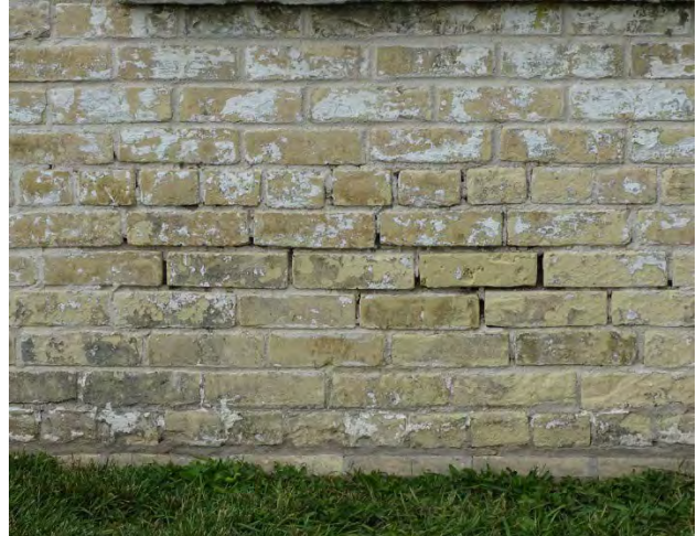
Figure No. 97: South Elevation (Photo No. 18.1)
