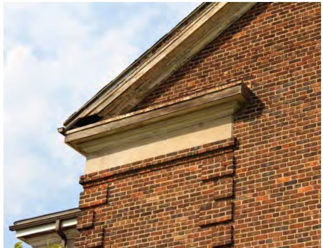
Figure No. 300: South Gable Detail (Photo No. 11.3)
