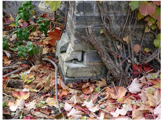
Figure No. 41: East Elevation – Sanctuary South Pier Base Detail (Photo No. 21.11)
