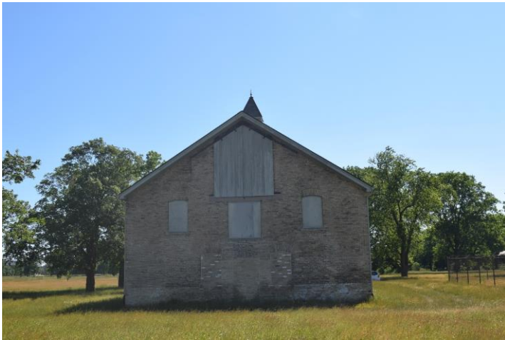
Photo 3: Horse Stable west elevation looking east
