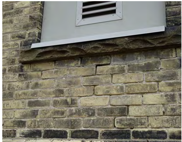
Figure No. 187: Central Administration Block – West Elevation (Photo No. 81.1)
