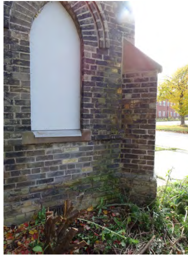
Figure No. 47: North Elevation – West/Main Entrance (Photo No. 20.4)
