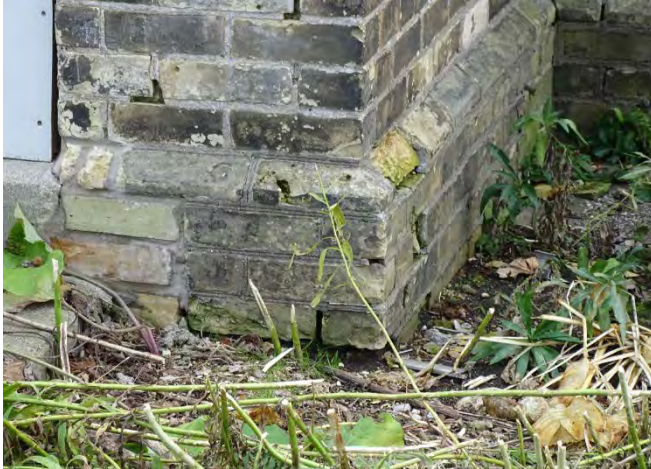
Figure No. 44: North Elevation – North Transept (Photo No. 20.9)
