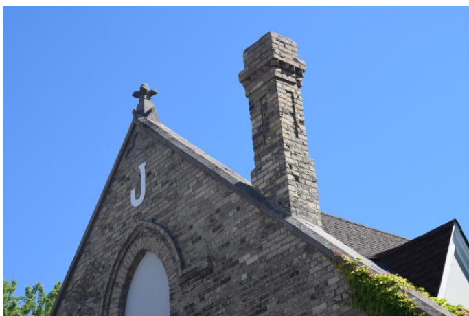
Photo 23: Chapel of Hope close-up of west elevation chimney
