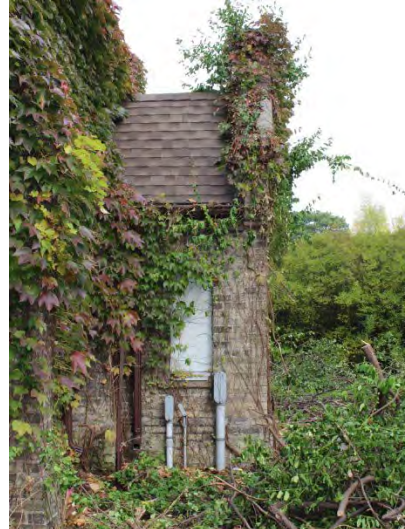
Figure No. 11: West Elevation – South Transept (Photo No. 8.2)
