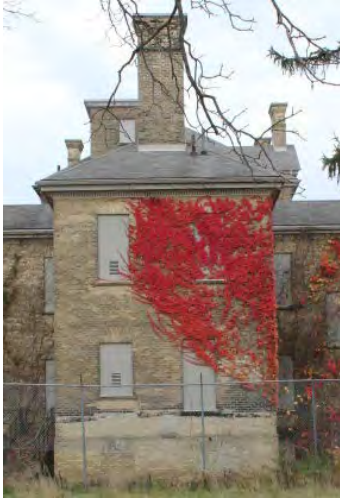
Figure No. 172: Central Pavilion – Chimney – North Elevation (Photo No. 73.0)
