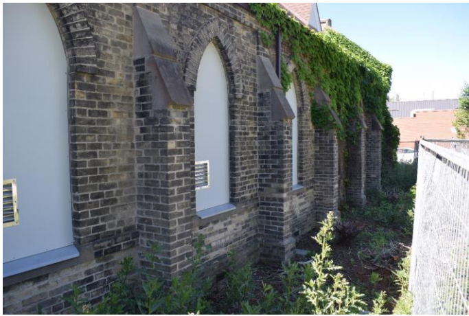
Photo 25: Chapel of Hope buttresses on south elevation looking east
