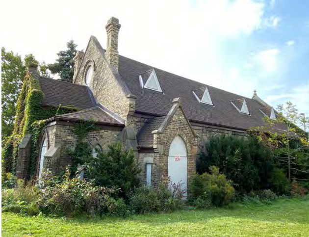
Figure No. 6: North Roof Shingles (Photo No. 5.0)
