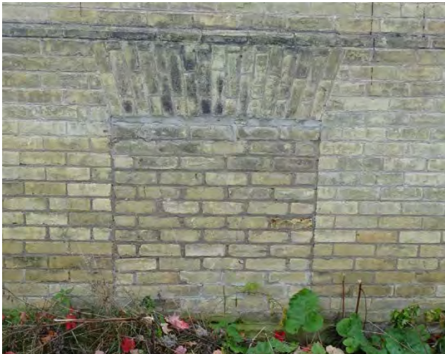
Figure No. 190: Central Pavilion and Corridors – Pavilion – North Elevation (Photo No. 82.1)
