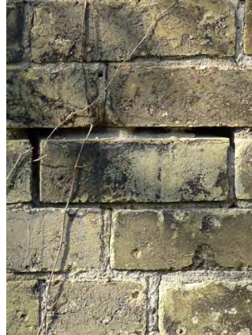
Figure No. 39: East Elevation – North Entrance Wing Brick Detail (Photo No. 21.6)
