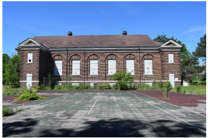
Photo 56: Recreation Hall east elevation looking west
