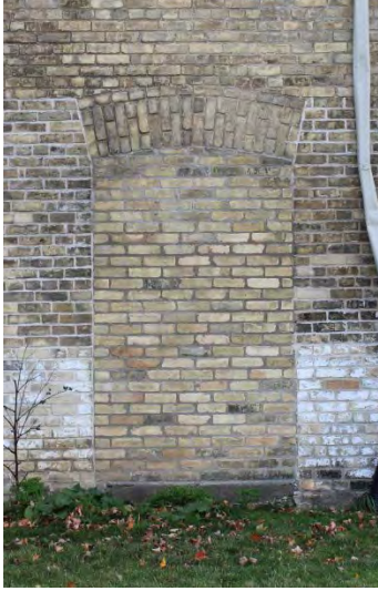
Figure No. 118: Door N-D1 (Photo No. 25.0)
