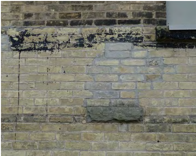
Figure No. 192: Central Pavilion and Corridors – Pavilion – North Elevation (Photo No. 82.3)
