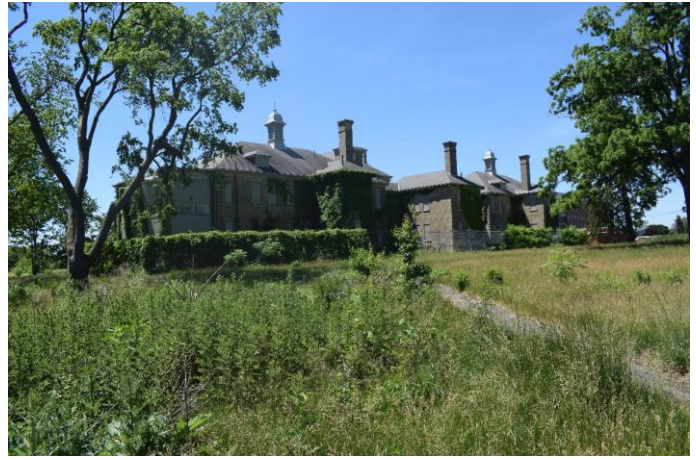
Photo 32: Infirmery north (rear) elevation looking southwest
