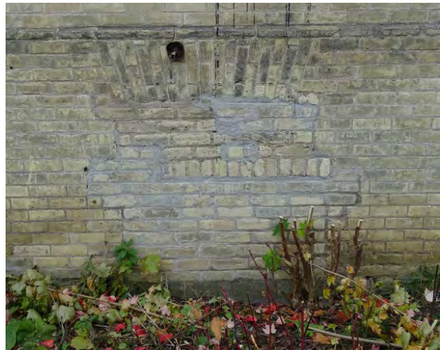
Figure No. 191: Central Pavilion and Corridors – Pavilion – North Elevation (Photo No. 82.2)
