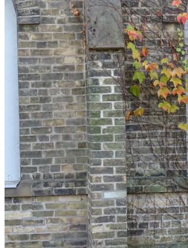
Figure No. 33: North Elevation – Previous Mortar Replacement (Photo No. 20.3)
