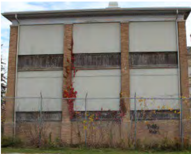
Figure No. 224: West Wing – West Porches – West Elevation (Photo No. 104.0)
