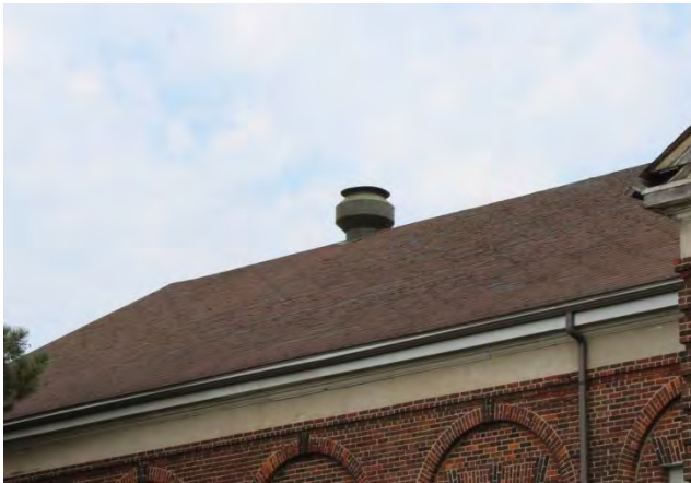
Figure No. 285: West Elevation Main Roof (Photo No. 8.1)
