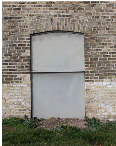
Figure No. 121: Door S-D3 (Photo No. 25.3)
