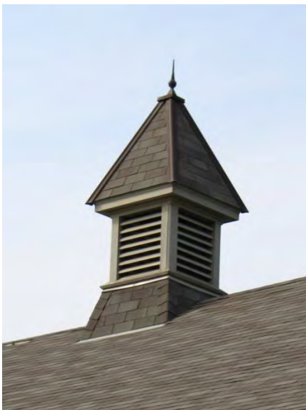
Figure No. 80: Ventilator (Photo No. 15.0)
