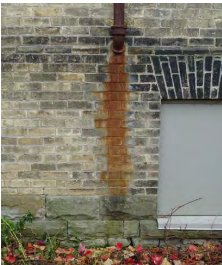
Figure No. 204: West Wing – North Elevation (Photo No. 86.2)
