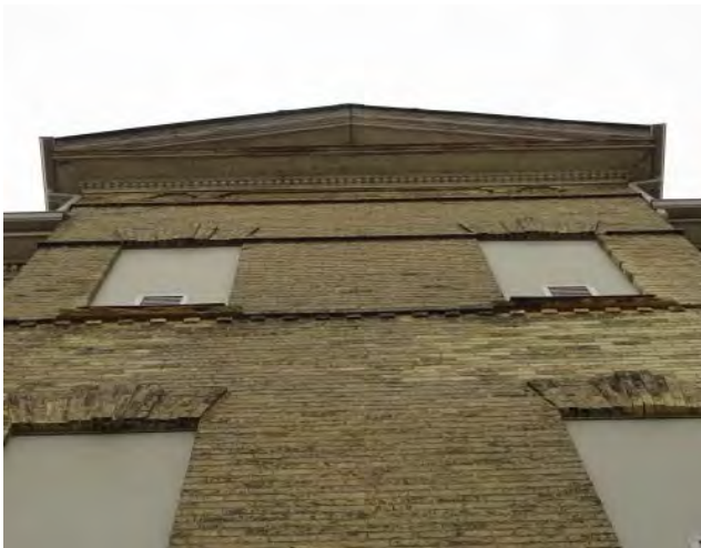
Figure No. 186: Central Administration Block – West Elevation – Frontispiece (Photo No. 81.0)
