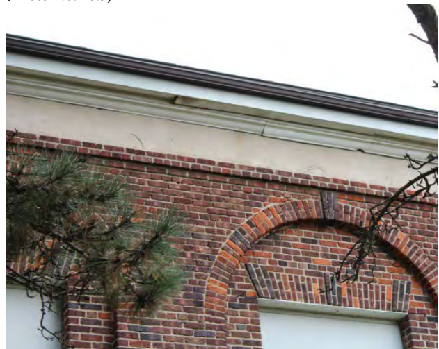
Figure No. 296: West Elevation Main Roof (Centre) (Photo No. 12.4)
