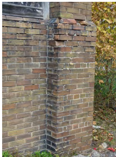
Figure No. 219: East Wing – East Porches – South Elevation (Photo No. 102.8)
