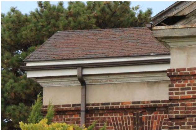
Figure No. 287: South Elevation Rear West Wing Roof (Photo No. 7.2)
