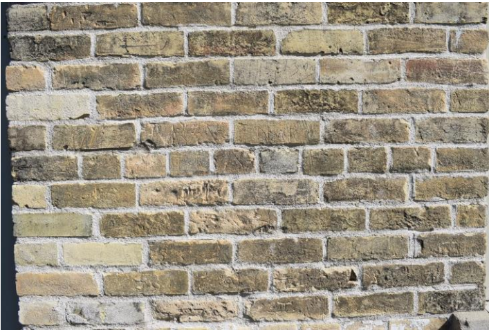
Photo 9: Horse Stable close-up of brick
