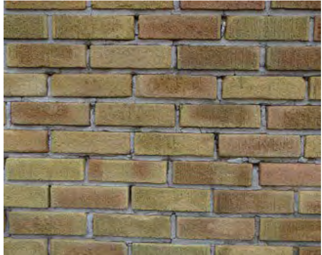
Figure No. 275: Central Administration Block – Entrance – West Elevation – Detail (Photo No. 108.5)
