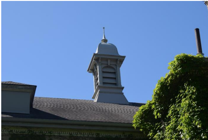
Photo 39: Infirmary close-up of ventilator looking southwest
