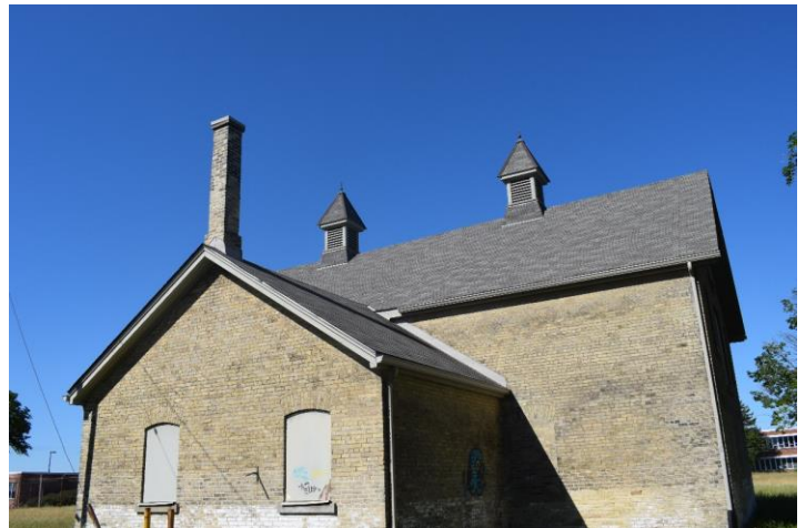
Photo 6: Horse Stable east elevation looking southwest
