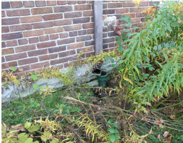
Figure No. 311: East Elevation at Grade (Photo No. 14.2)
