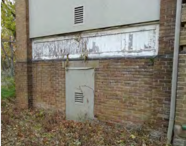
Figure No. 214: East Wing – East Porches – North Elevation (Photo No. 100.1)
