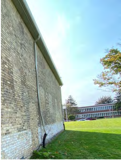
Figure No. 86: North Elevation RWL (Photo No. 11.0)
