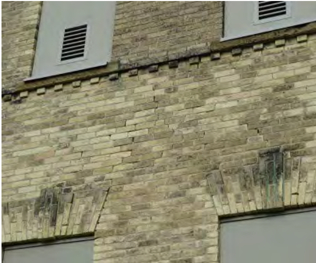
Figure No. 196: East Wing – South Elevation (Photo No. 85.4)
