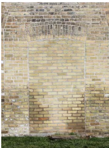
Figure No. 122: Door W-D1 (Photo No. 25.4)
