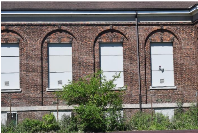
Photo 63: Recreation Hall east elevation boarded-up windows with venting
