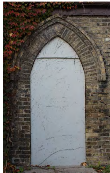
Figure No. 66: Door E-D1 (Photo No. 33.1)
