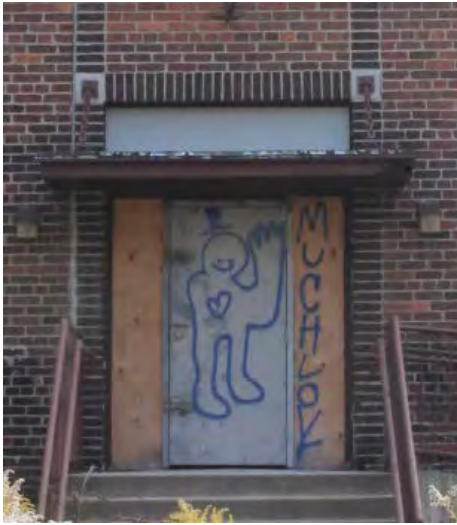
Figure No. 339: Door N-D1 (Photo No. 27.0)
