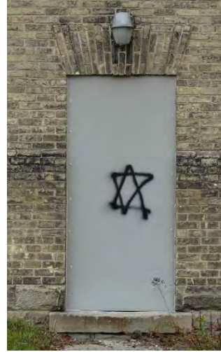
Figure No. 271: West Wing – South Elevation (Photo No. 107.9)
