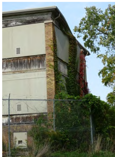
Figure No. 217: East Wing – East Porches – East Elevation (Photo No. 101.1)
