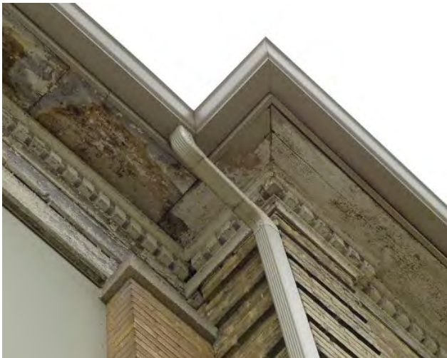
Figure No. 152: West Wing – East Elevation Detail (Photo No. 52.13)
