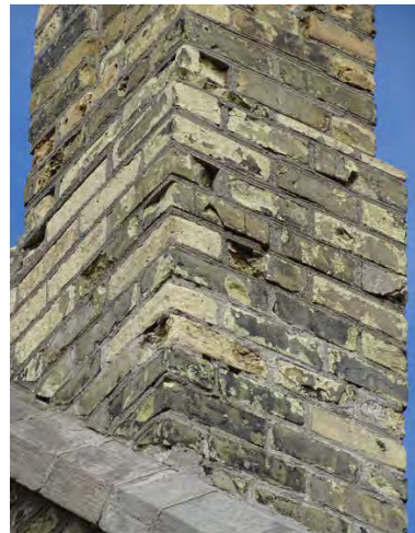
Figure No. 31: West Gable – South Chimney – Detail (Photo No. 19.5)
