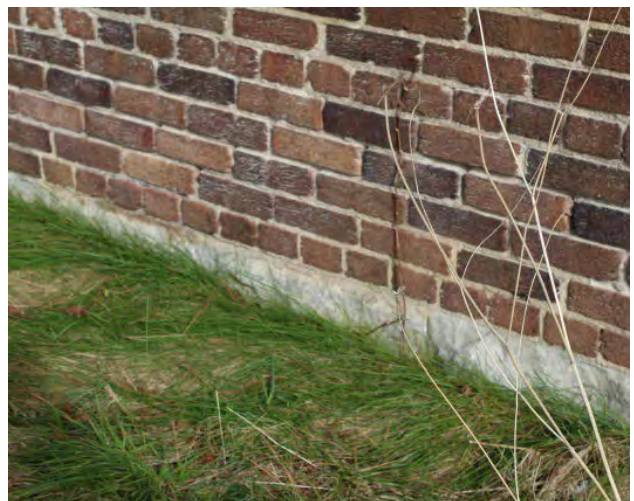
Figure No. 328: West Elevation Foundation (Photo No. 25.0)
