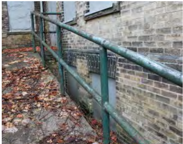
Figure No. 279: Central Pavilion and Corridors (Photo No. 109.6)
