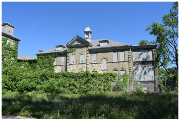
Photo 30: Infirmary south elevation of east wing looking north
