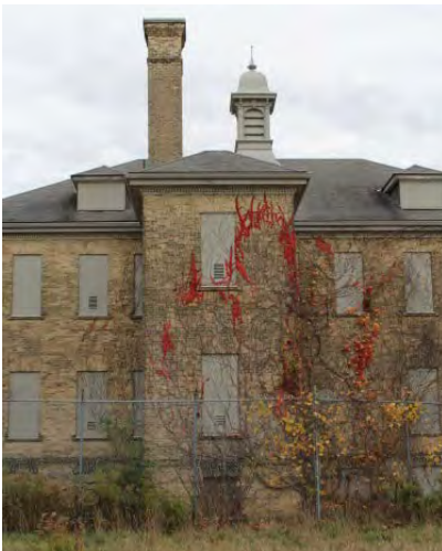
Figure No. 176: West Wing – Stair Tower Chimney – North Elevation (Photo No. 75.0)
