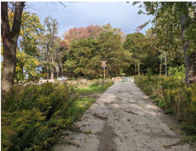
Figure No. 377: View to south of railway crossing with barricades, west road (Photo No. 7.10)
