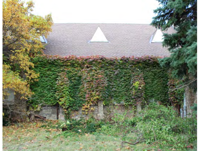
Figure No. 7: South Roof Shingles (Photo No. 7.0)
