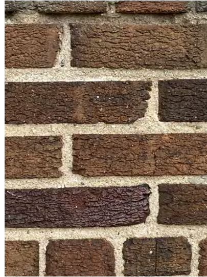
Figure No. 318: Typical Brick Coursing and Mortar (Photo No. 19.4)
