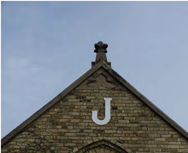
Figure No. 73: West Elevation – West/Main Entrance – Letter "J" (Photo No. 34.0)
