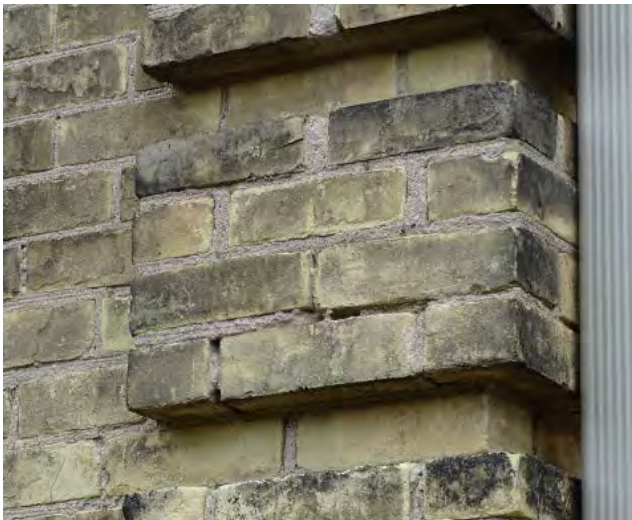
Figure No. 202: West Wing – North Elevation (Photo No. 86.4)
