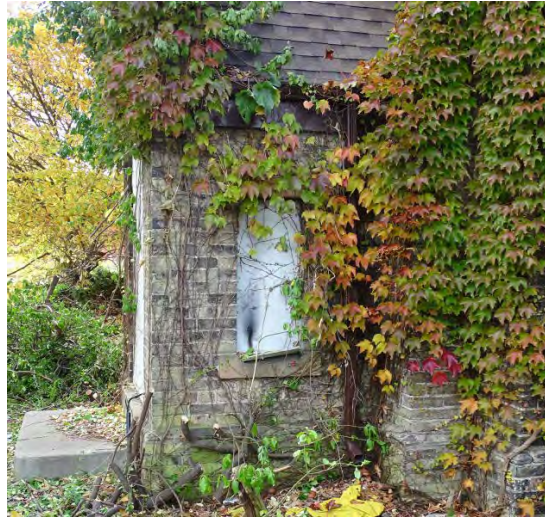
Figure No. 23: East Elevation – South Transept Gutter and RWL (Photo No. 14.4)
