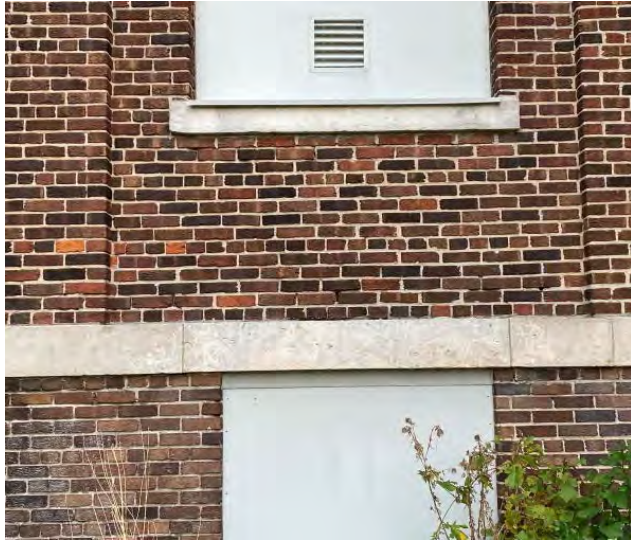
Figure No. 317: East Elevation Stone Band Detail (Photo No. 19.1)
