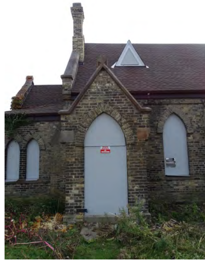
Figure No. 43: North Elevation – North Transept (Photo No. 20.7)
