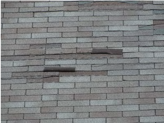
Figure No. 78: South Elevation Shingles Detail (Photo No. 6.3)
