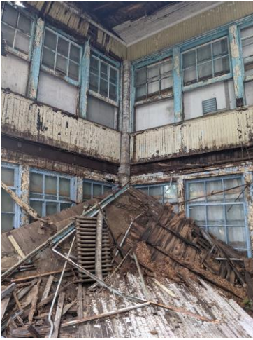
Photo 49: Infirmary east porch roof collapse, photo provided by Old Oak from June 25, 2021
