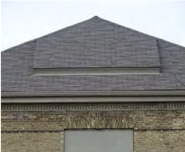
Figure No. 128: Central Administration Block – South Elevation – Skylight Detail (Photo No. 23.1)
