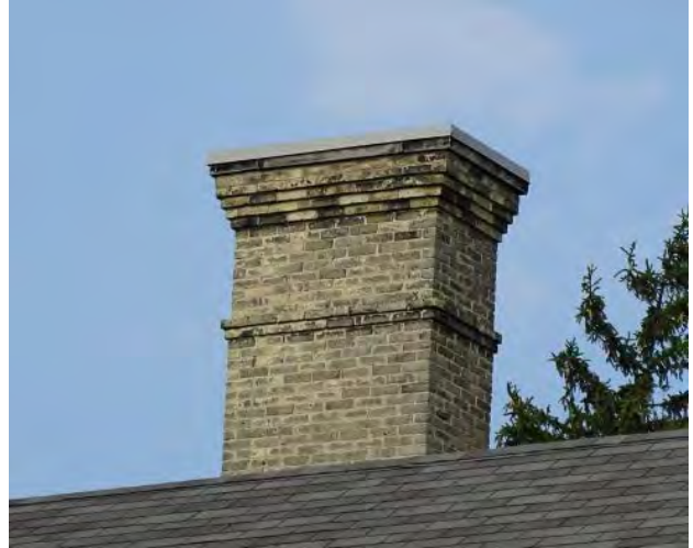
Figure No. 173: Central Pavilion – Chimney – South East Elevation Detail (Photo No. 73.3)
