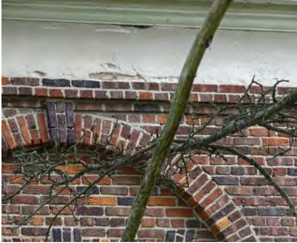
Figure No. 297: West Elevation Main Roof (Centre) (Detail) (Photo No. 12.5)
