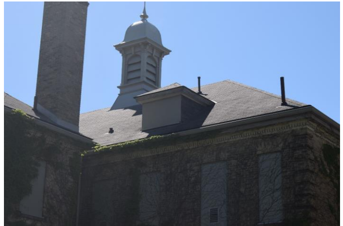
Photo 40: Infirmary close-up of dormer on West Wing looking southwest
