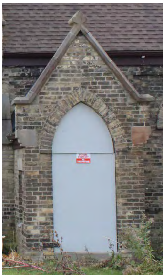
Figure No. 65: Door N-D1 (Photo No. 33.0)
