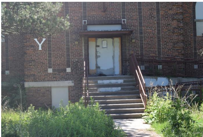
Photo 65: Recreation Hall front elevation entry door, staircase and ramp looking south
