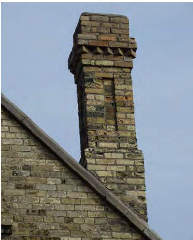
Figure No. 30: West Gable – South Chimney – West Elevation (Photo No. 19.2)
