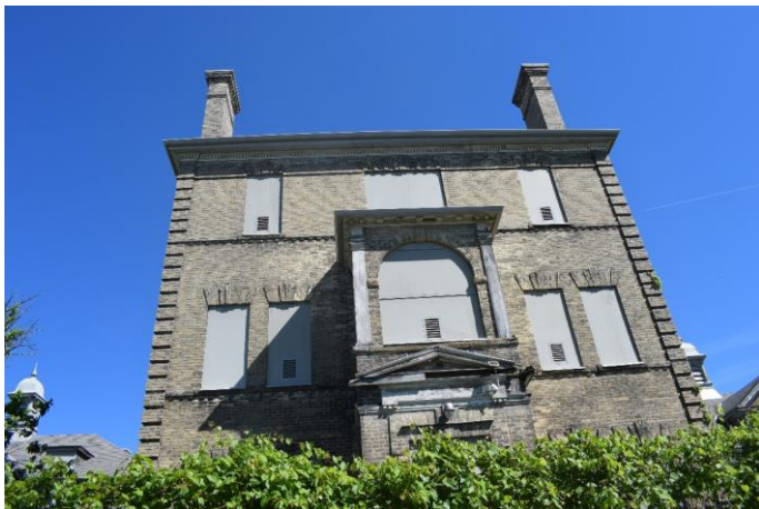
Photo 27: Infirmary south elevation of Administration Block looking north
