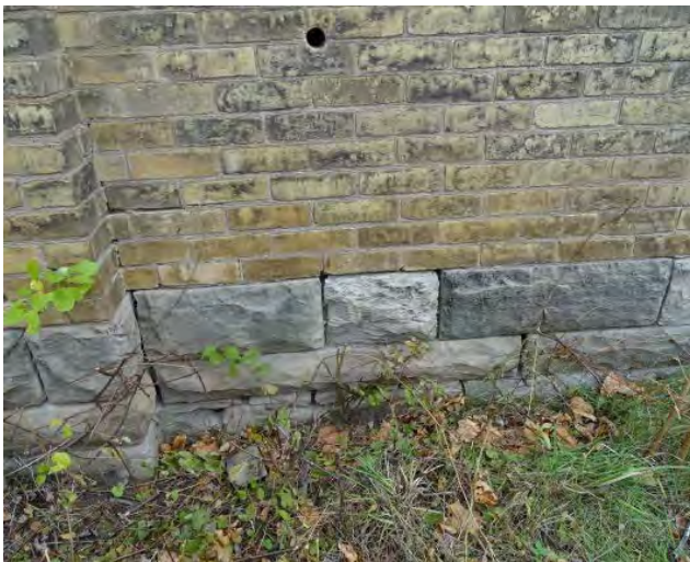
Figure No. 206: Central Administration Block – West Elevation (Photo No. 90.2)
