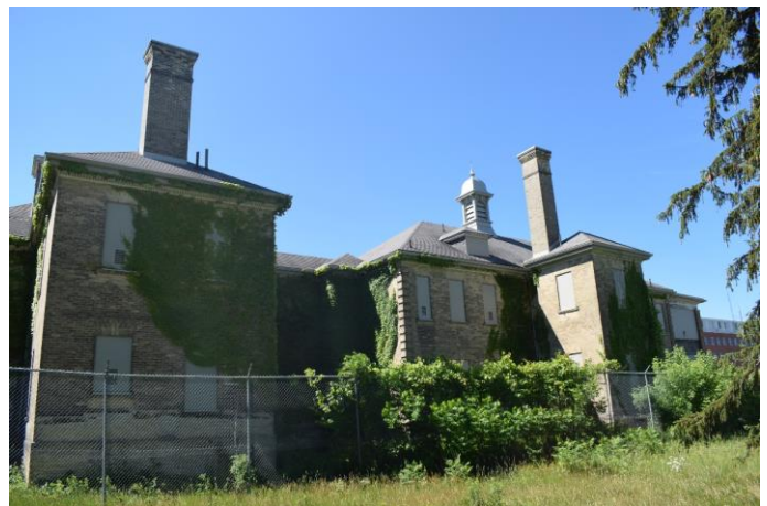
Photo 36: Infirmery rear elevation of central pavilion and west wing looking southwest
