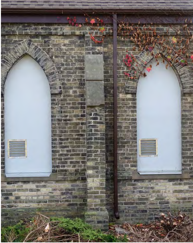
Figure No. 16: North Elevation – Main Roof RWL (Photo No. 13.1)
