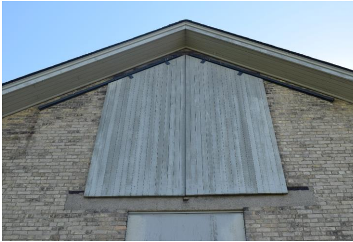
Photo 13: Horse Stable west elevation boarded-up hay loft door
