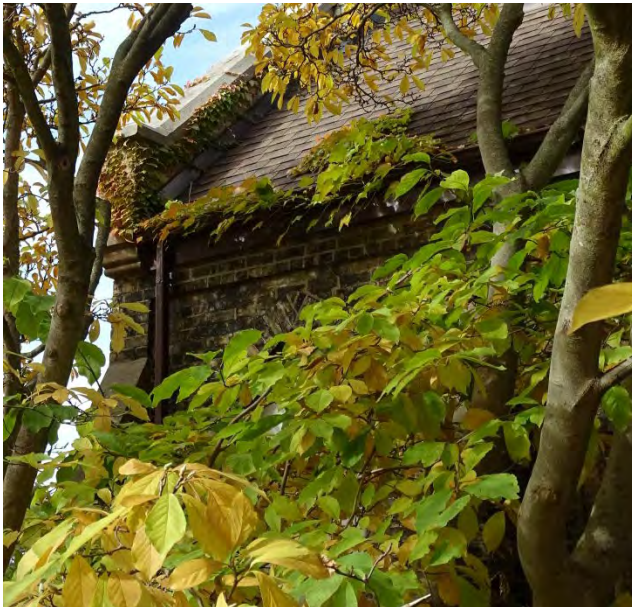
Figure No. 18: South Elevation – Main Roof Gutter and RWL (Photo No. 15.1)
