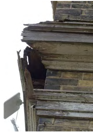
Figure No. 139: Central Administration Block – East Elevation – Entrance Detail (Photo No. 41.8)
