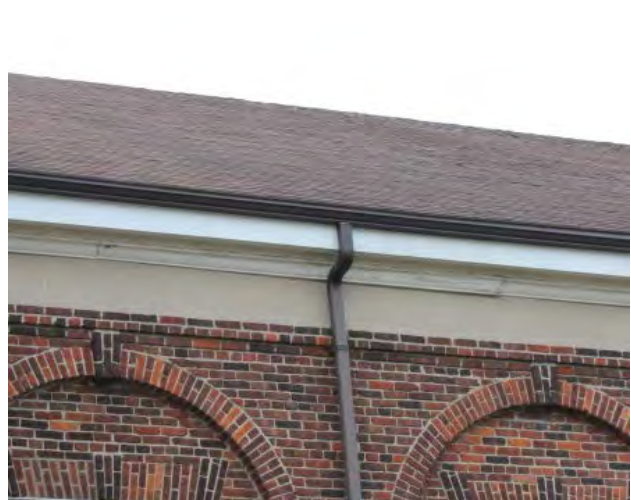
Figure No. 294: East Elevation Main Roof (Centre) Detail (Photo No. 10.5)
