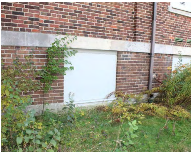
Figure No. 327: East Elevation Foundation (Photo No. 23.0)
