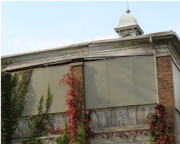
Figure No. 216: East Wing – East Porches – East Elevation (Photo No. 101.3)
