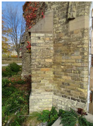
Figure No. 49: West Elevation – West/Main Entrance North Brick Pier (Photo No. 23.5)
