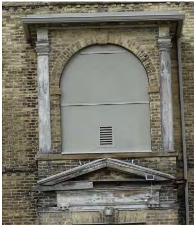
Figure No. 138: Central Administration Block – Entrance – South Elevation (Photo No. 41.1)
