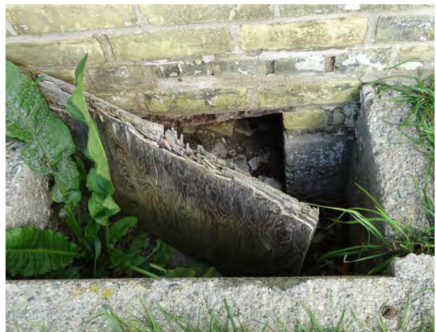
Figure No. 101: West Elevation Detail (Photo No. 23.1)
