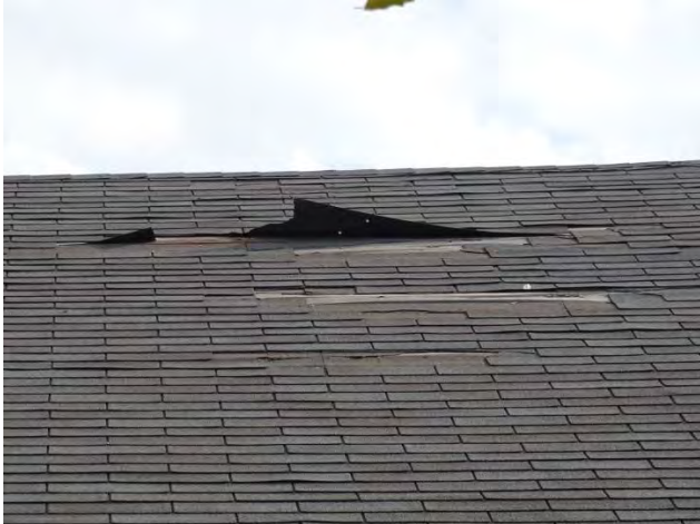
Figure No. 76: North Elevation Shingles Detail (Photo No. 5.2)
