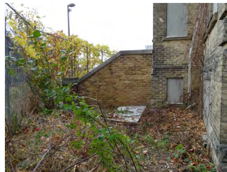
Figure No. 273: Central Administration Block – Entrance – East Elevation (Photo No. 108.1)
