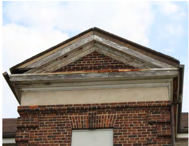
Figure No. 306: Rear West Wing West Pediment (Photo No. 12.7)
