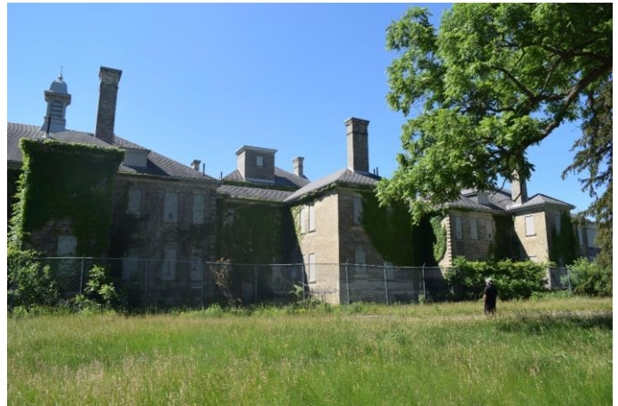
Photo 34: Infirmery rear elevation of east wing and central pavilion looking southwest
