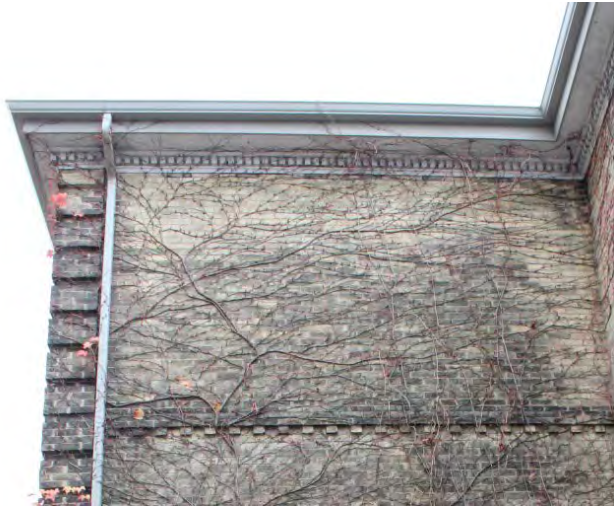
Figure No. 150: West Wing – East Elevation Detail (Photo No. 51.3)
