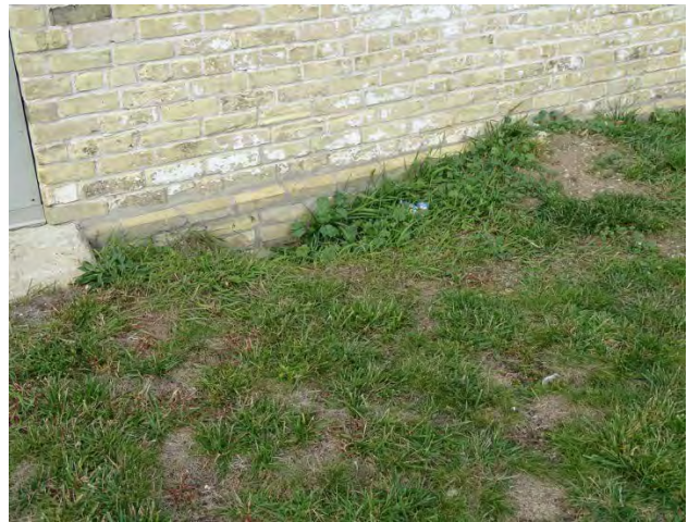
Figure No. 99: South Elevation (Photo No. 22.2)
