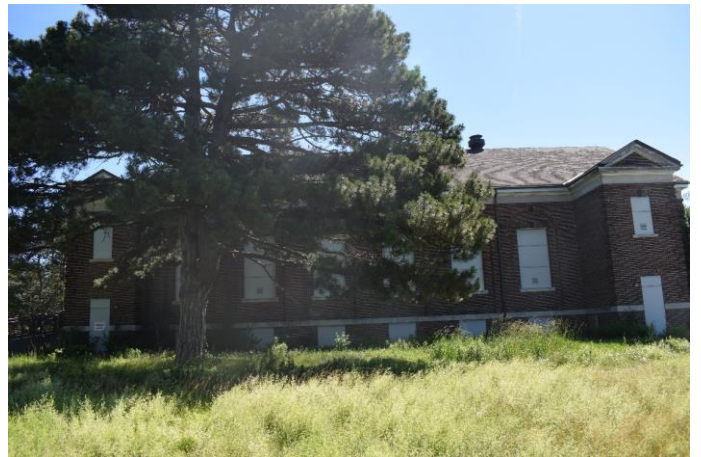
Photo 54: Recreation Hall west elevation looking east
