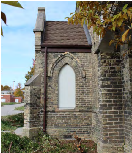
Figure No. 48: South Elevation – West/Main Entrance (Photo No. 22.1)
