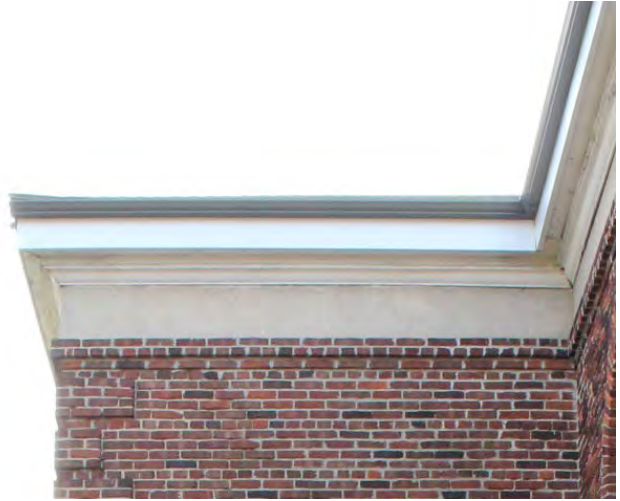
Figure No. 304: Rear East Wing East Pediment North Return (Photo No. 9.5)
