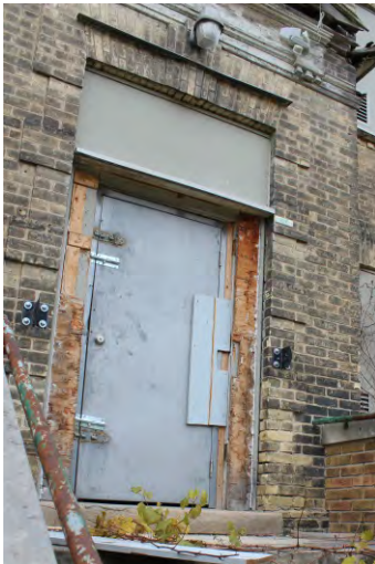
Figure No. 262: Central Administration Block – Entrance – South Elevation – D1-S (Photo No. 107.0)
