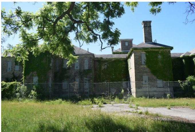
Photo 35: Infirmery rear elevation of east wing and central pavilion looking south
