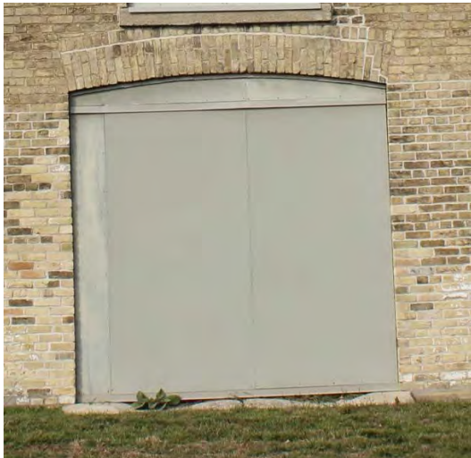
Figure No. 120: Door S-D2 (Photo No. 25.2)
