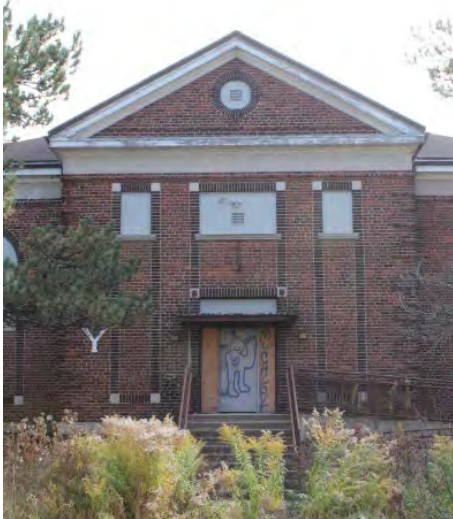
Figure No. 315: North Elevation Frontispiece, Front Entrance (Photo No. 18.0)
