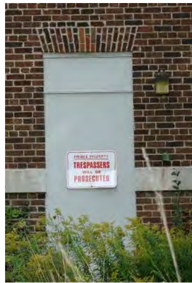
Figure No. 342: Door W-D1 (Photo No. 27.3)
