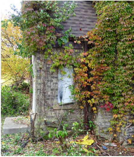
Figure No. 46: East Elevation – North Transept (Photo No. 21.15)
