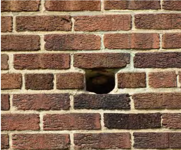
Figure No. 323: South Gable Penetration in Masonry (Photo No. 20.2)
