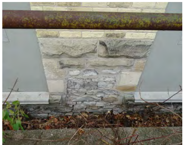
Figure No. 213: East Wing – South Elevation (Photo No. 94.2)
