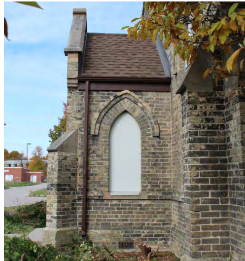
Figure No. 25: South Elevation – West/Main Entrance Gutter RWL (Photo No. 15.0)
