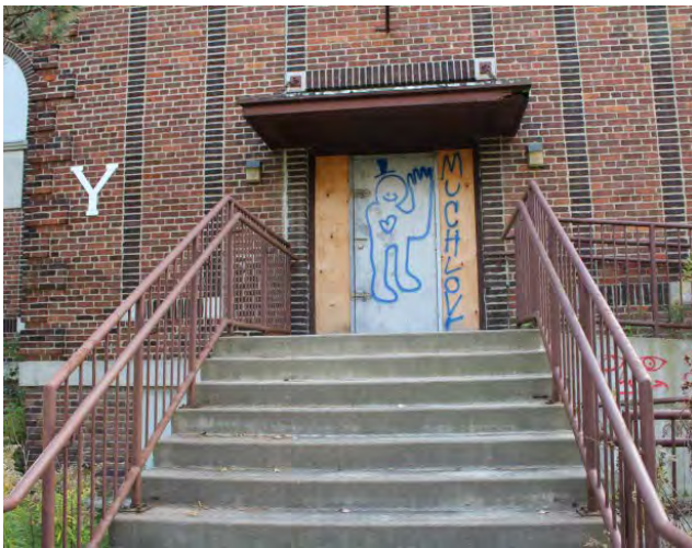
Figure No. 348: North Elevation, Stairs (Photo No. 29.0)
