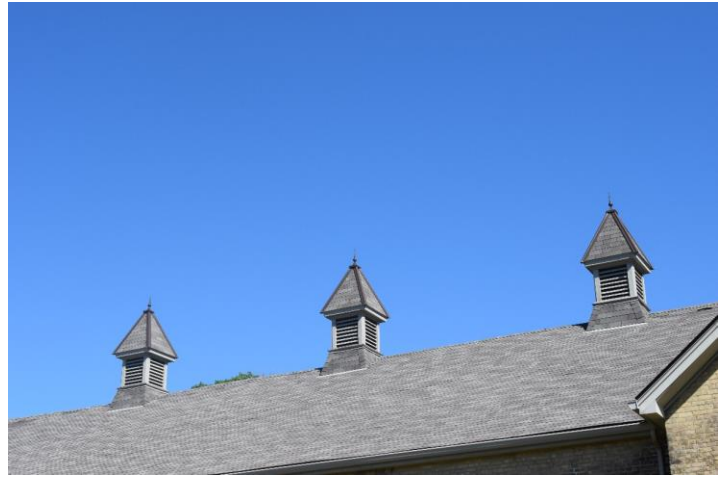
Photo 8: Horse Stable north elevation view of ventilators looking southeast
