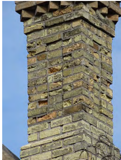
Figure No. 29: East Gable – South East Chimney – Detail (Photo No. 18.4)
