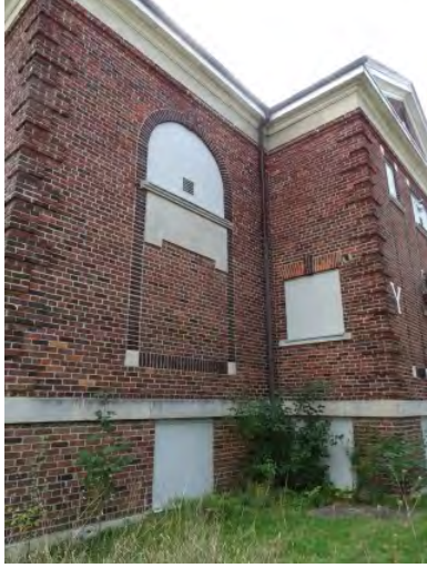
Figure No. 309: North Elevation Frontispiece East Wing (Photo No. 13.0)
