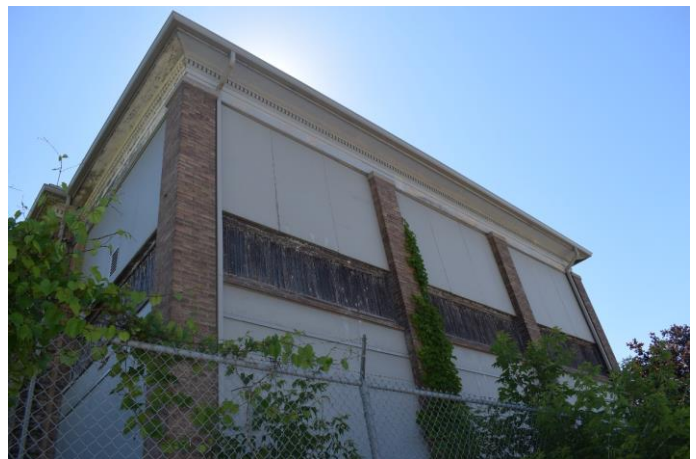
Photo 42: Infirmary close-up of dentilated cornice on west elevation porch end
