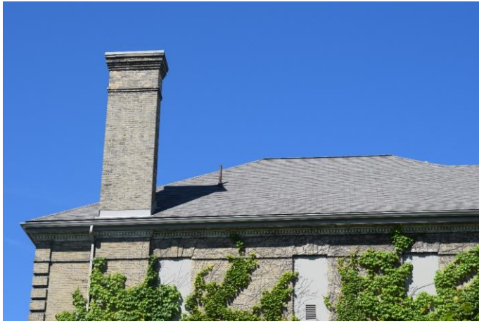
Photo 37: Close-up of Administration Block chimney looking southwest
