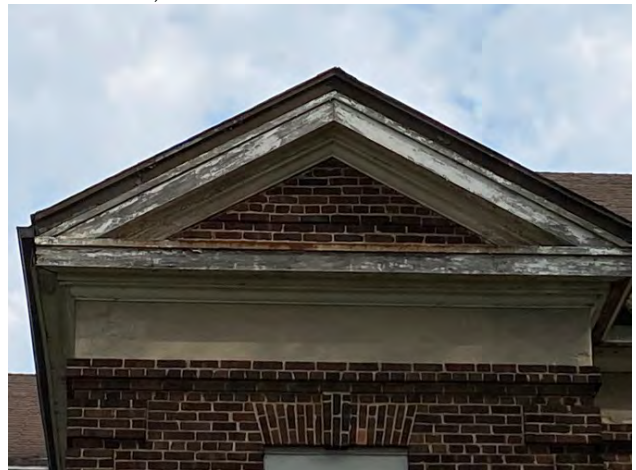
Figure No. 308: Frontispiece West Wing West Pediment (Photo No. 12.1)
