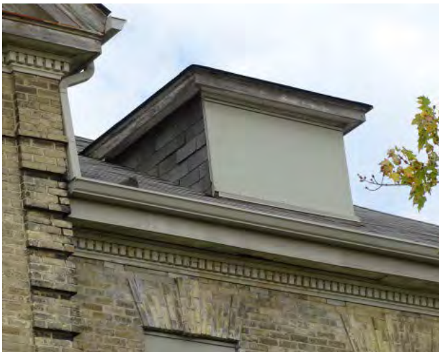
Figure No. 180: West Wing – South Elevation – South East Dormer (Photo No. 77.3)
