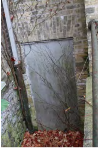
Figure No. 270: West Wing – Stair Tower – East Elevation (Photo No. 107.8)
