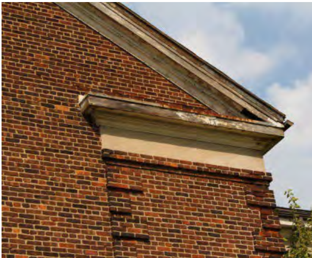
Figure No. 299: South Gable Detail (Photo No. 11.2)
