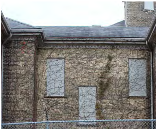
Figure No. 130: East Corridor– North Elevation (Photo No. 25.1)
