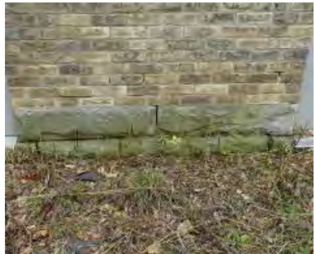
Figure No. 207: Central Administration Block – West Elevation (Photo No. 90.0)
