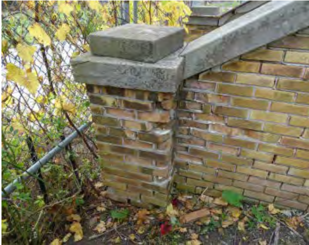
Figure No. 274: Central Administration Block – Entrance – East Elevation – Detail (Photo No. 108.2)
