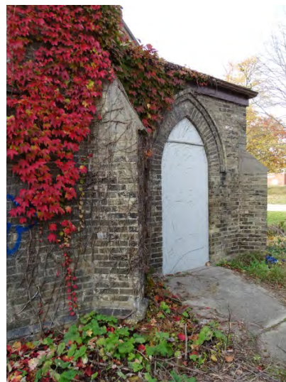
Figure No. 37: East Elevation – Sanctuary North Pier (Photo No. 21.7)
