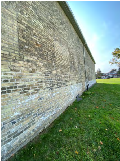
Figure No. 94: North Elevation (Photo No. 20.0)
