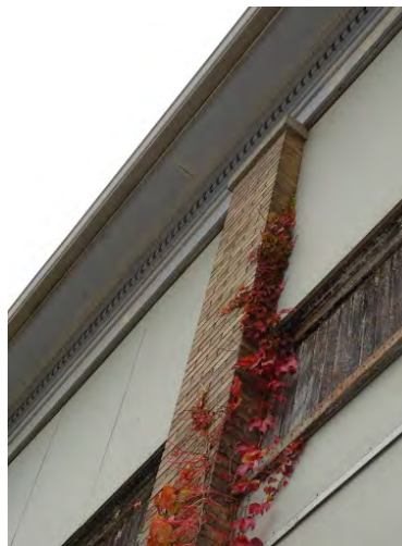
Figure No. 153: West Wing – East Elevation Detail (Photo No. 53.1)
