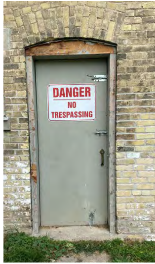
Figure No. 119: Door S-D1 (Photo No. 25.1)
