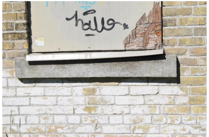
Photo 12: Horse Stable close-up of window sill
