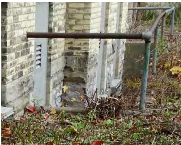
Figure No. 212: East Wing – South Elevation (Photo No. 94.0)
