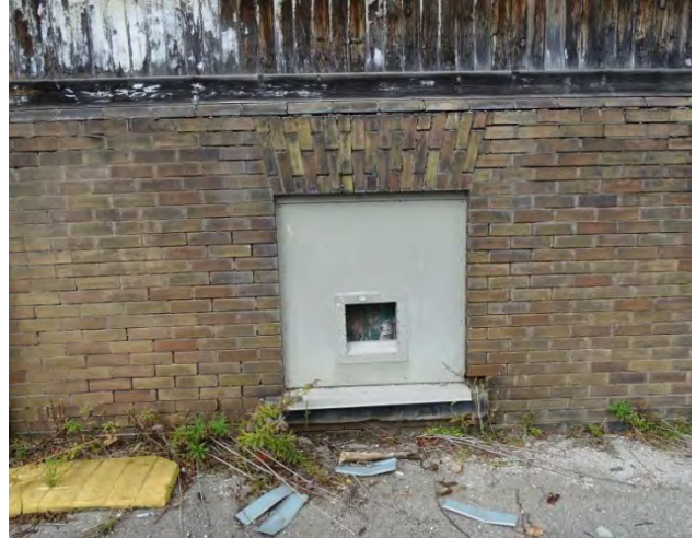
Figure No. 215: East Wing – East Porches – South Elevation (Photo No. 102.5)
