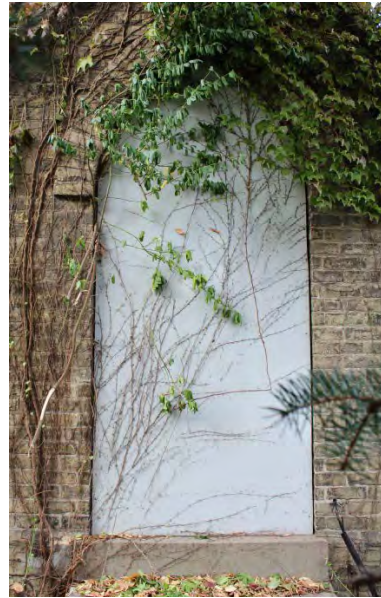
Figure No. 68: Door S-D1 (Photo No. 33.3)
