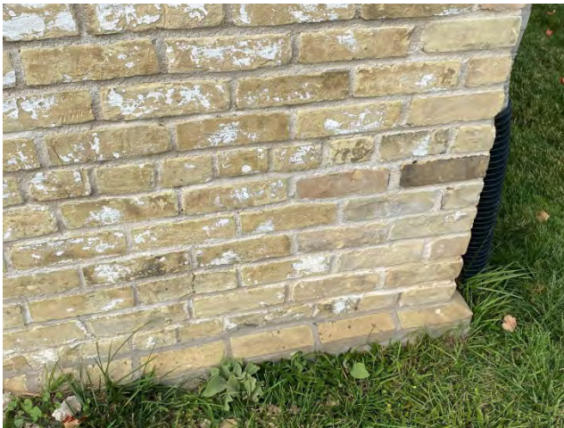
Figure No. 98: South Elevation (Photo No. 22.1)
