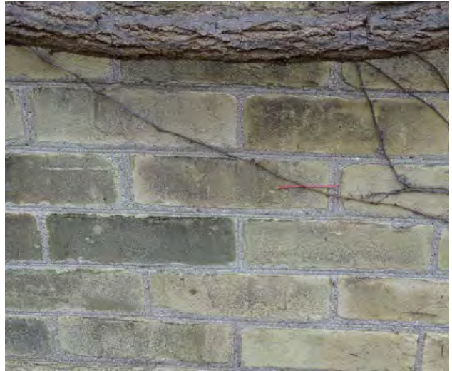
Figure No. 201: West Wing – North Elevation (Photo No. 86.1)
