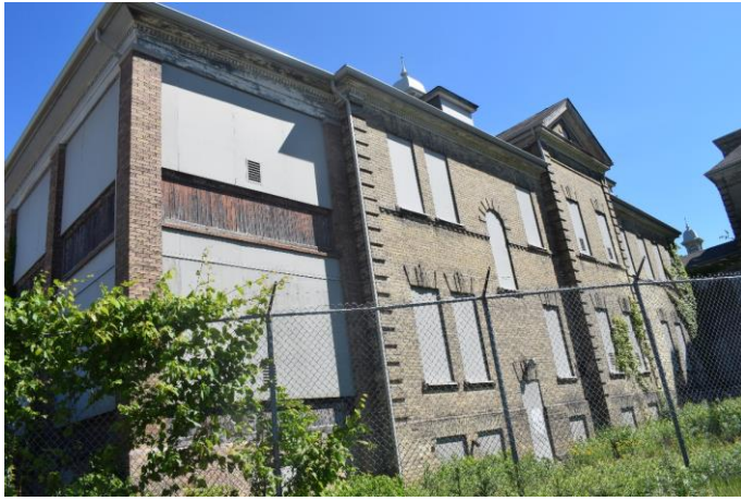
Photo 31: Infirmery south elevation of west wing looking northeast
