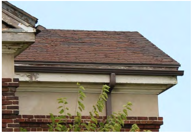
Figure No. 286: South Elevation Rear East Wing Roof (Photo No. 7.1)
