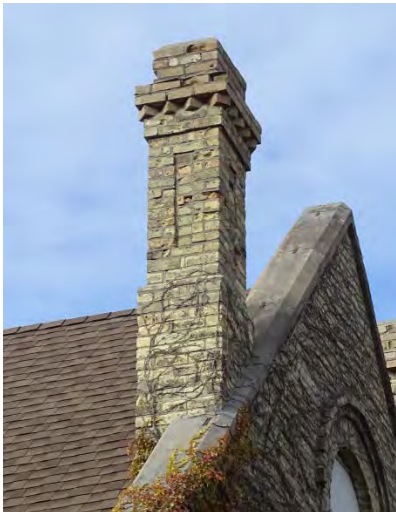
Figure No. 28: East Gable – South Chimney – South Elevation (Photo No. 18.2)
