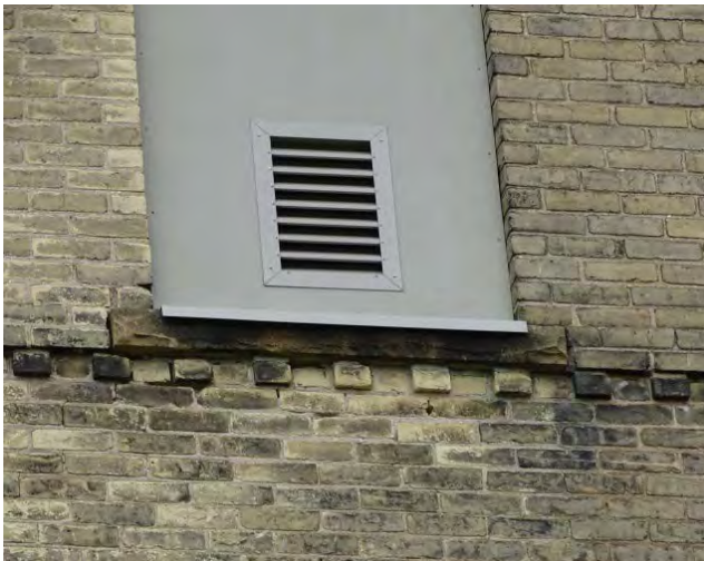
Figure No. 184: Central Administration Block – South Elevation – Detail (Photo No. 80.2)
