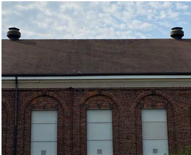
Figure No. 313: Ventilator (Photo No. 17.0)
