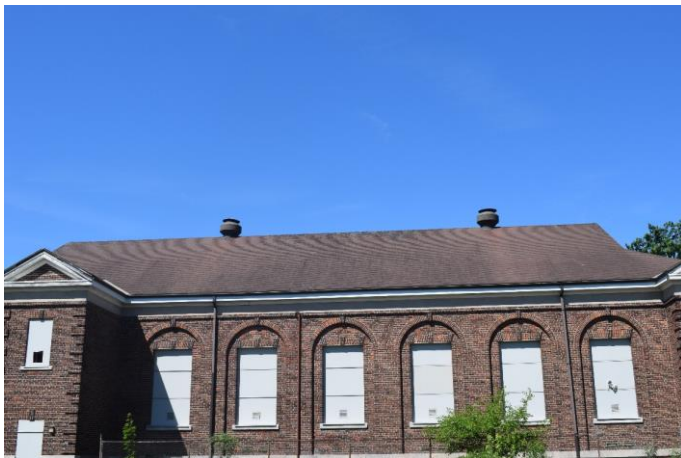
Photo 57: Recreation Hall east elevation roof looking west
