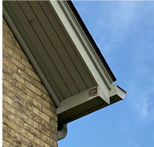
Figure No. 83: West Elevation Soffit Detail (Photo No. 10.0)
