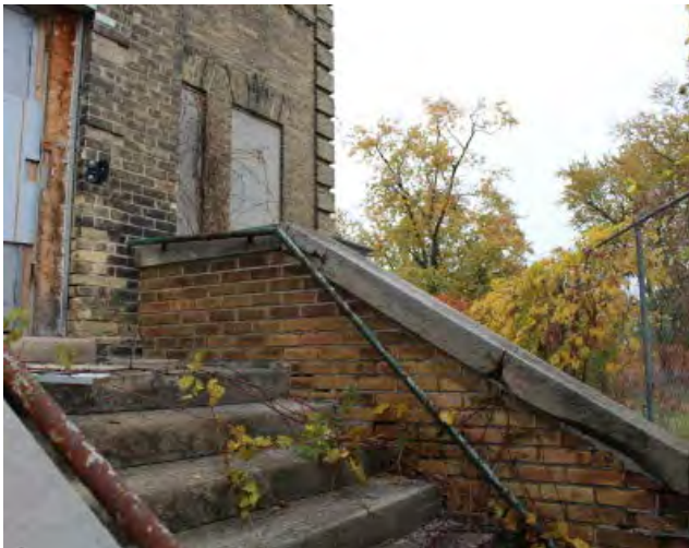
Figure No. 276: Central Administration Block – Entrance – West Elevation (Photo No. 108.7)
