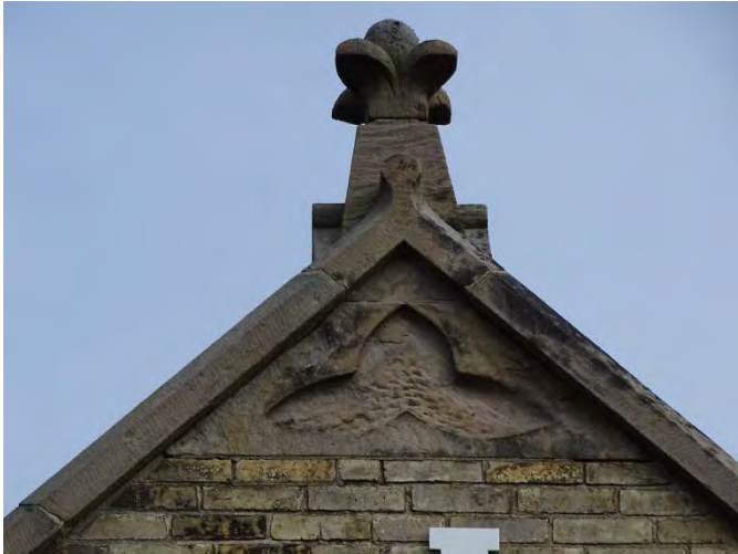
Figure No. 50: West Elevation – West Gable Stone Detailing (Photo No. 27.2)
