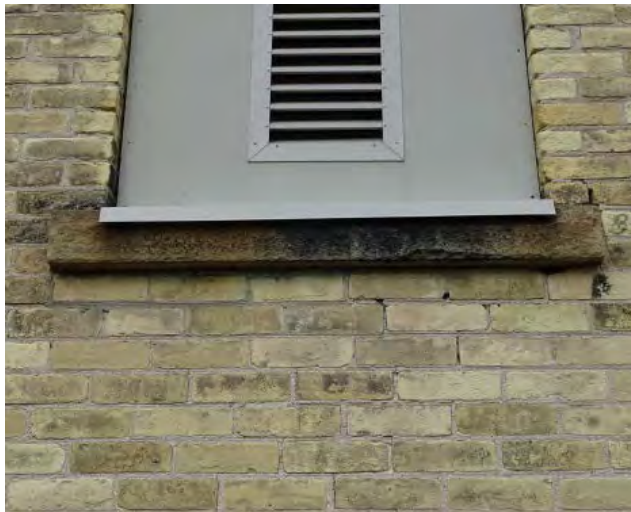
Figure No. 260: Stained Sill Detail (Photo No. 106.34)
