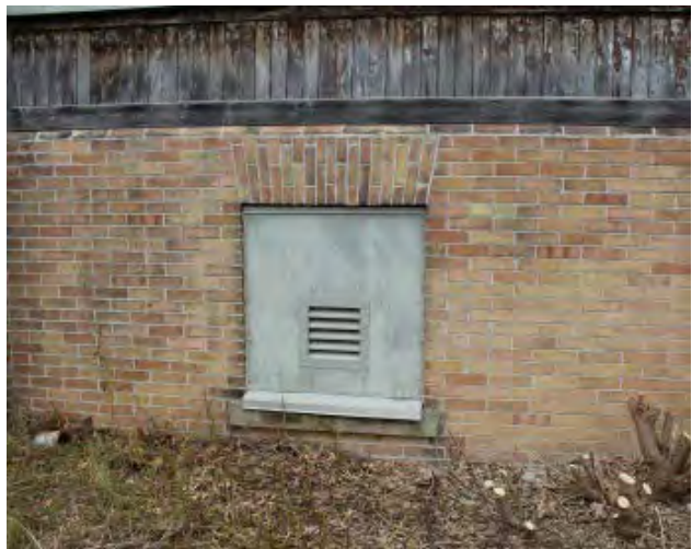
Figure No. 223: West Wing – West Porches – South Elevation (Photo No. 105.2)
