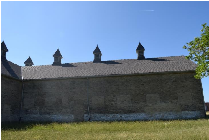
Photo 5: Horse Stable north elevation looking south
