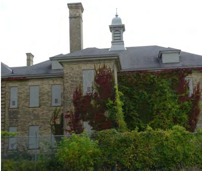
Figure No. 162: West Wing – North Elevation (Photo No. 79.0)
