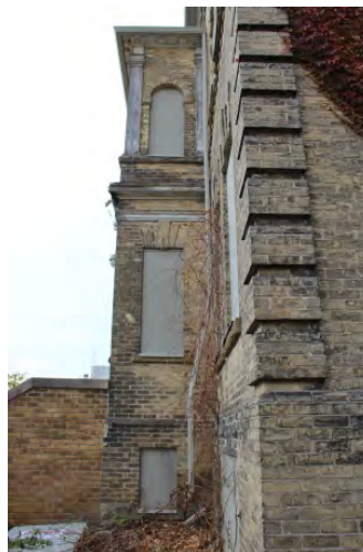
Figure No. 155: Central Administration Block – Entrance – East Elevation (Photo No. 56.1)
