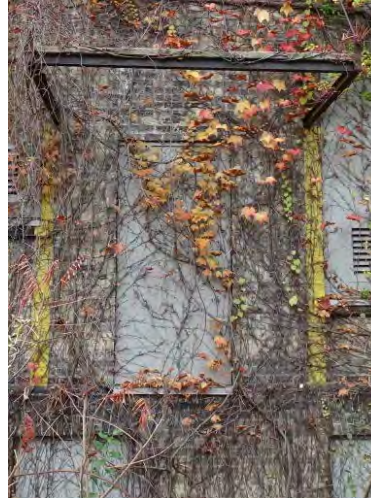
Figure No. 265: Central Administration Block – East Elevation – D3-E (Photo No. 107.3)
