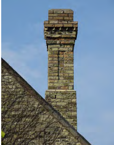
Figure No. 26: East Gable – North Chimney – East Elevation (Photo No. 17.1)
