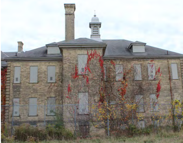
Figure No. 136: West Wing – North Elevation (Photo No. 33.0)
