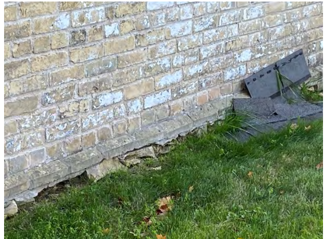
Figure No. 95: North Elevation Foundation (Photo No. 20.1)
