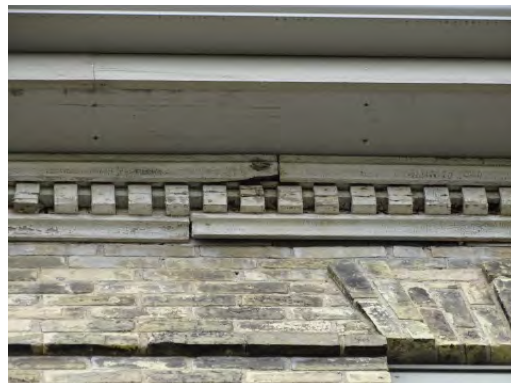
Figure No. 141: Central Administration Block – South Elevation Detail (Photo No. 39.3)
