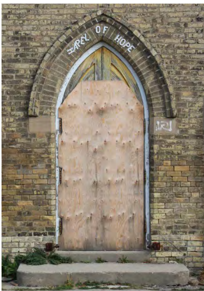
Figure No. 71: Door W-D1 (Photo No. 33.6)
