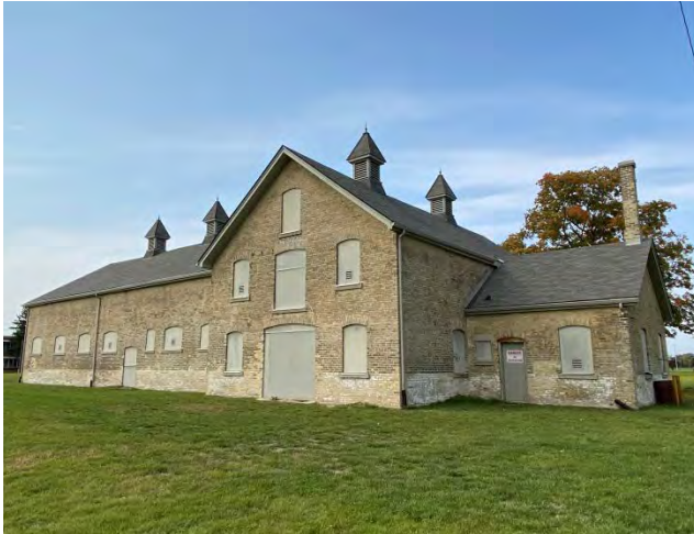
Figure No. 96: South Elevation (Photo No. 18.0)
