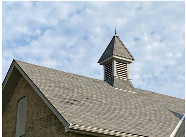
Figure No. 79: West Elevation, North Gable (Photo No. 6.5)
