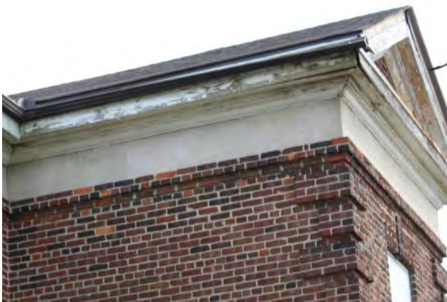
Figure No. 307: Rear West Wing West Pediment North Return (Photo No. 9.6)
