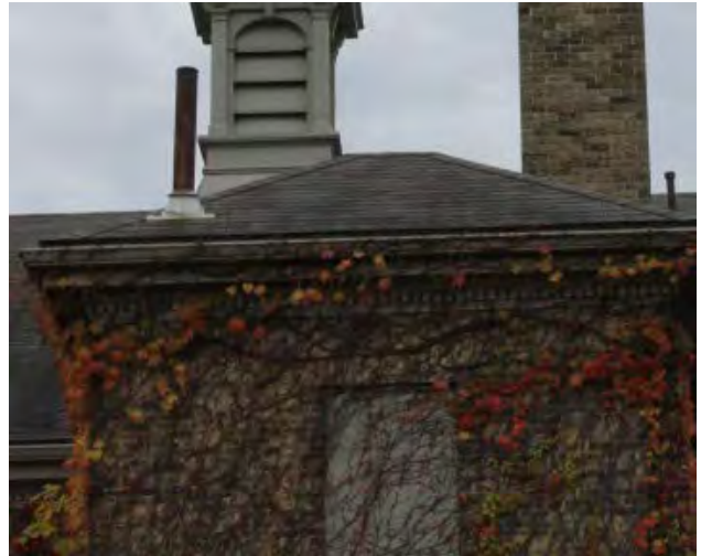
Figure No. 145: East Wing – Stair Tower – North Elevation (Photo No. 46.4)
