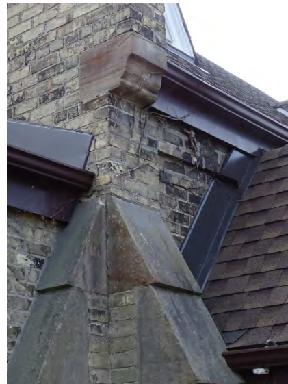
Figure No. 13: North Elevation – North Transept Fascia (Photo No. 9.1)
