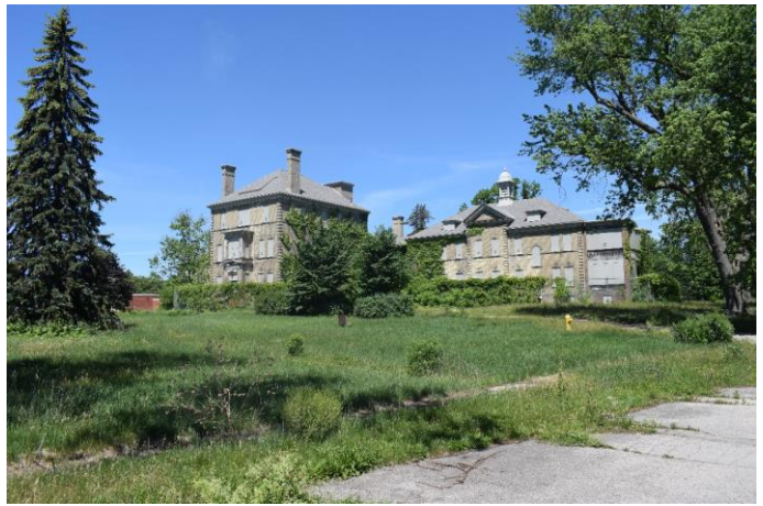
Photo 26: Infirmary south elevation looking northwest
