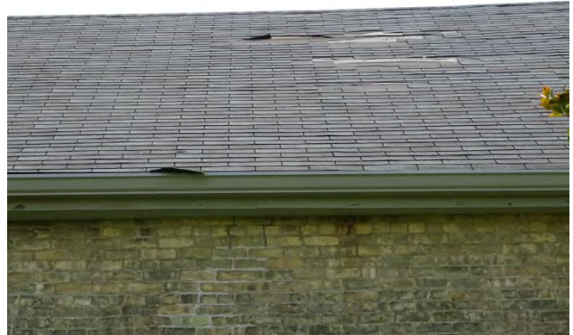
Figure No. 77: North Elevation Shingles Detail (Photo No. 5.3)
