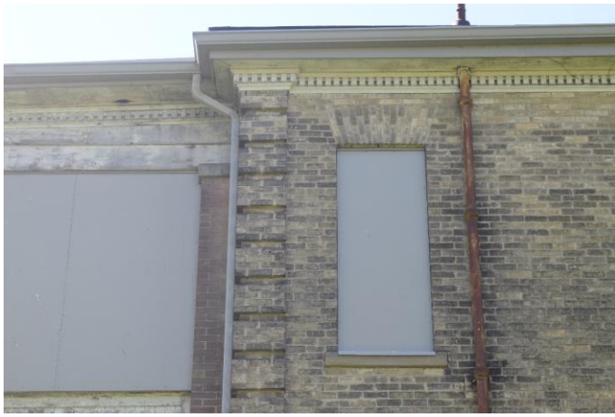
Photo 43: Infirmary close-up of window sill and brick voussoir on rear elevation of east wing
