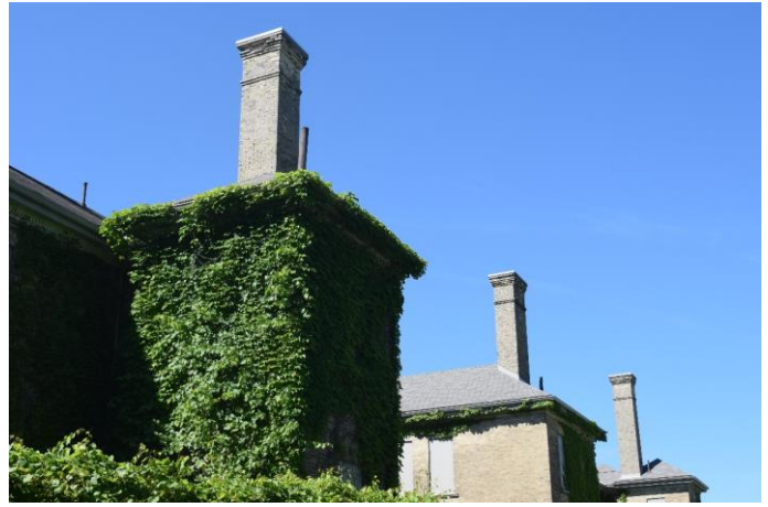
Photo 38: Infirmary rear elevation chimneys looking southwest
