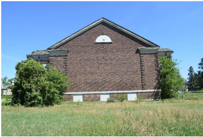
Photo 55: Recreation Hall south elevation looking north
