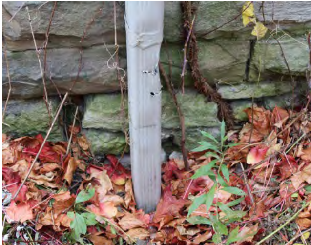
Figure No. 158: West Corridor – South Elevation – Detail at Grade (Photo No. 60.1)
