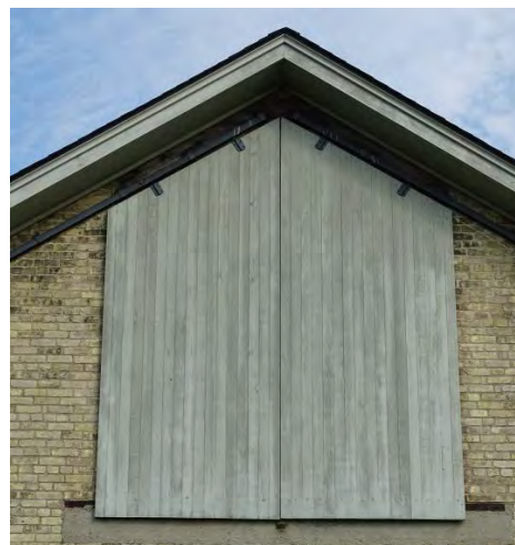
Figure No. 123: Door W-D2 – Hayloft Doors (Photo No. 25.5)
