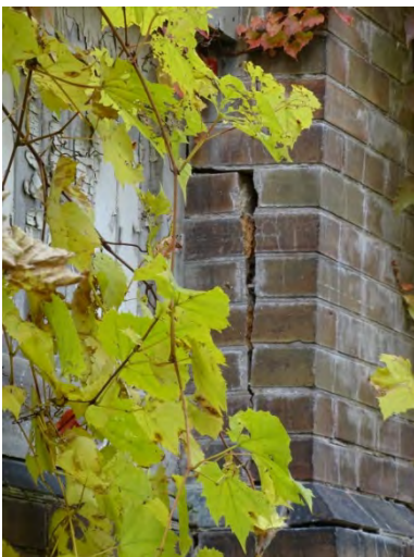
Figure No. 218: East Wing – East Porches – East Elevation (Photo No. 101.6)
