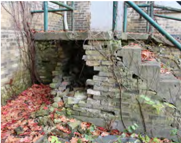
Figure No. 278: Central Pavilion and Corridors (Photo No. 109.3)
