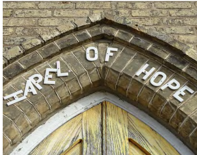
Figure No. 74: West Elevation – West/Main Entrance – "Chapel of Hope" (Photo No. 34.1)
