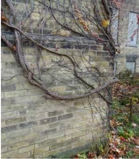
Figure No. 200: West Wing – North Elevation (Photo No. 86.0)
