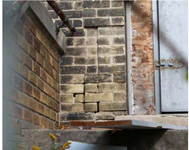
Figure No. 183: Central Administration Block – Entrance – South Elevation – Detail (Photo No. 80.1)
