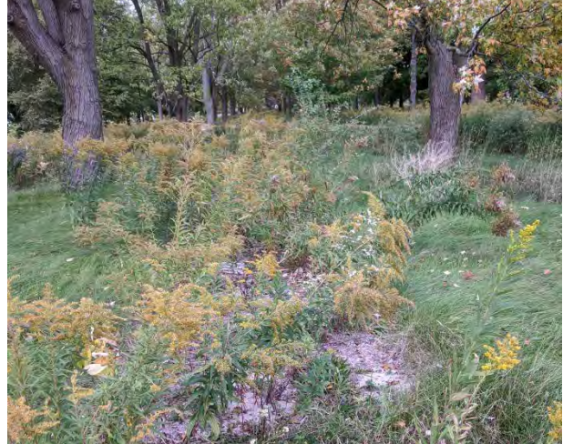
Figure No. 380: View to north along centre concrete walkway in poor condition (Photo No. 8.1)
