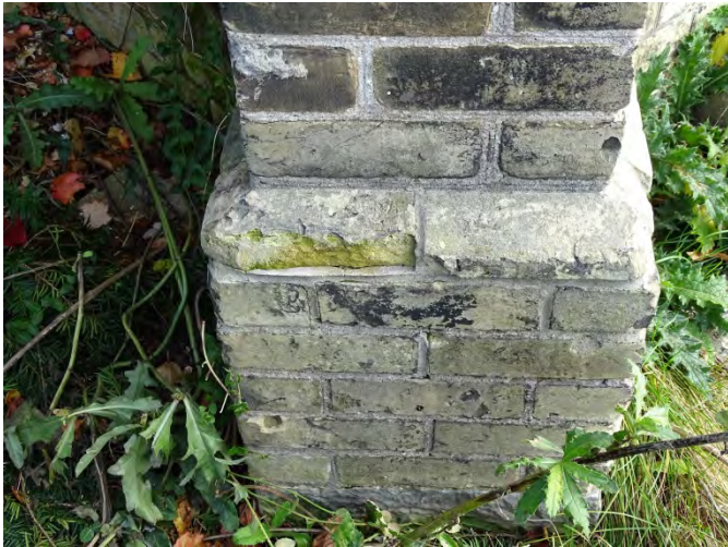
Figure No. 52: North Elevation – West/Main Entrance Exposed Stone Foundation (Photo No. 28.0)
