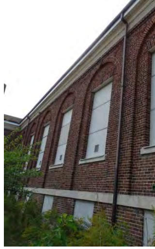
Figure No. 310: East Elevation (Photo No. 14.0)
