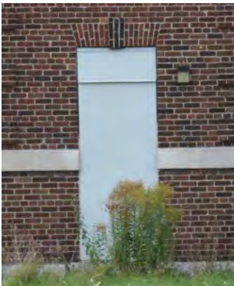
Figure No. 341: Door E-D2 (Photo No. 27.2)
