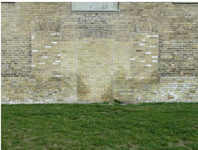
Figure No. 100: West Elevation (Photo No. 19.0)
