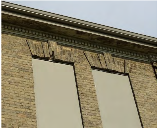
Figure No. 197: East Wing – South Elevation (Photo No. 85.5)
