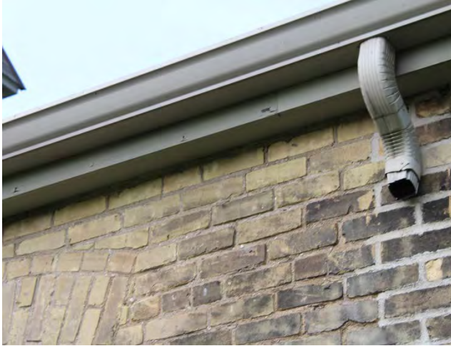
Figure No. 82: One Storey South Elevation Fascia (Photo No. 9.0)
