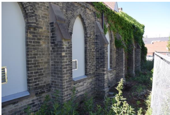
Photo 7: Chapel of Hope south elevation looking east
