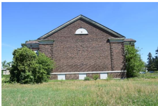
Photo 21: Recreation Hall south elevation looking north
