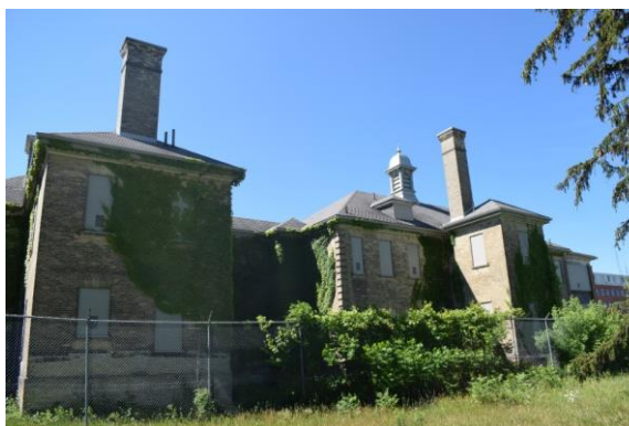
Photo 17: Infirmary rear elevation of central pavilion and west wing looking southwest
