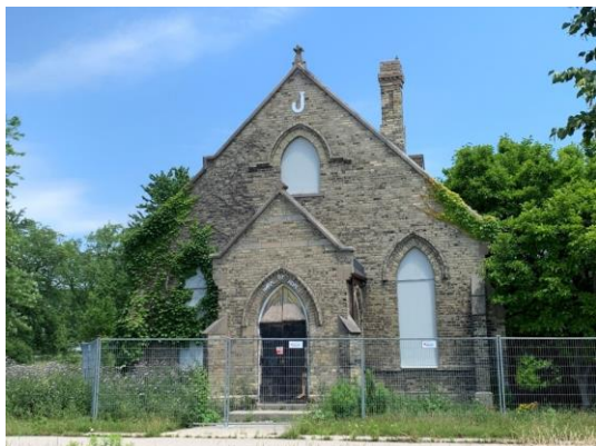
Photo 6: Chapel of Hope front (west) elevation looking northeast
