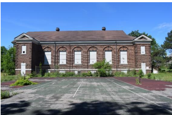
Photo 20: Recreation Hall east elevation looking west
