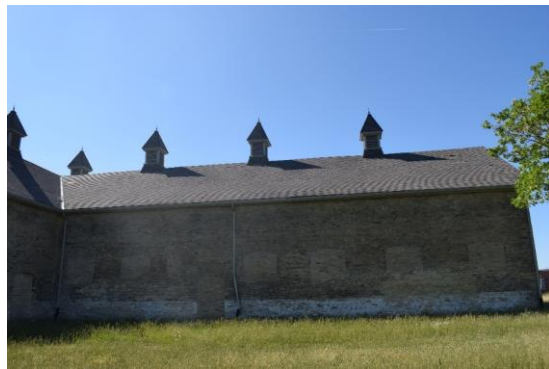
Photo 4: Horse Stable looking south
