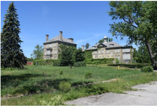
Photo 10: Infirmery south elevation looking northwest
