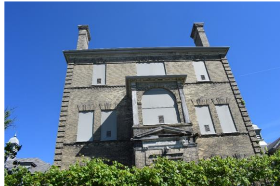
Photo 11: Infirmery south elevation of Administration Block looking north
