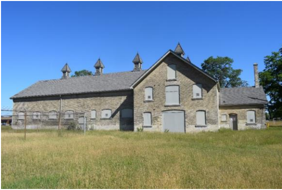
Photo 1: Horse Stable looking northwest
