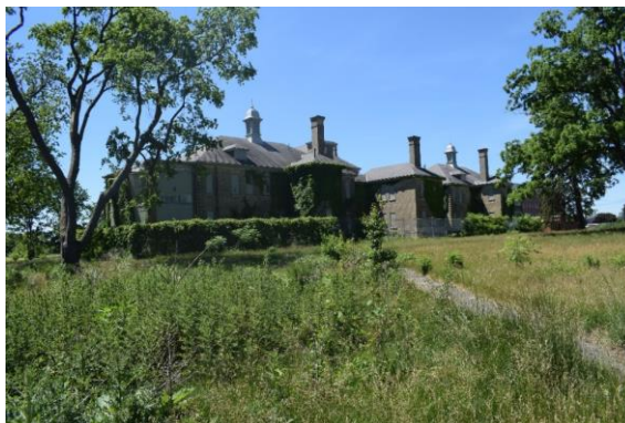
Photo 15: Infirmary north (rear) elevation looking southwest
