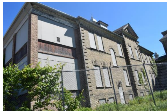
Photo 13: Infirmery south elevation of west wing looking northeast
