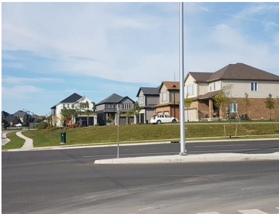
View to north/northeast at intersection of Bradley & Morgan
