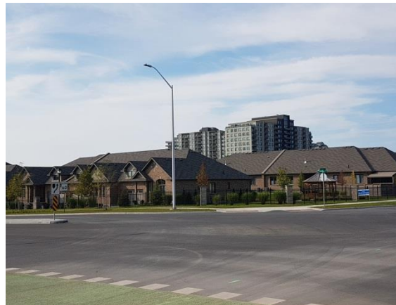
View to northwest at intersection of Bradley & Morgan
