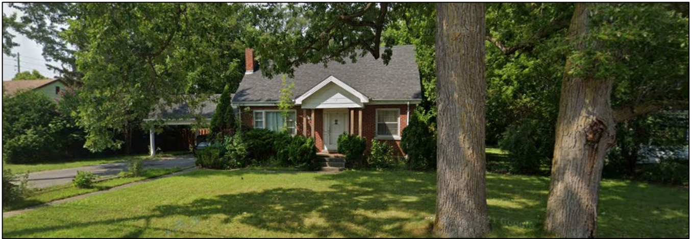
Photo 2. View of 417 Boler Road looking west from Boler Road.
