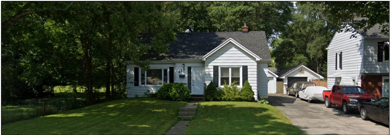
Photo 1. View of 415 Boler Road looking west from Boler Road.
