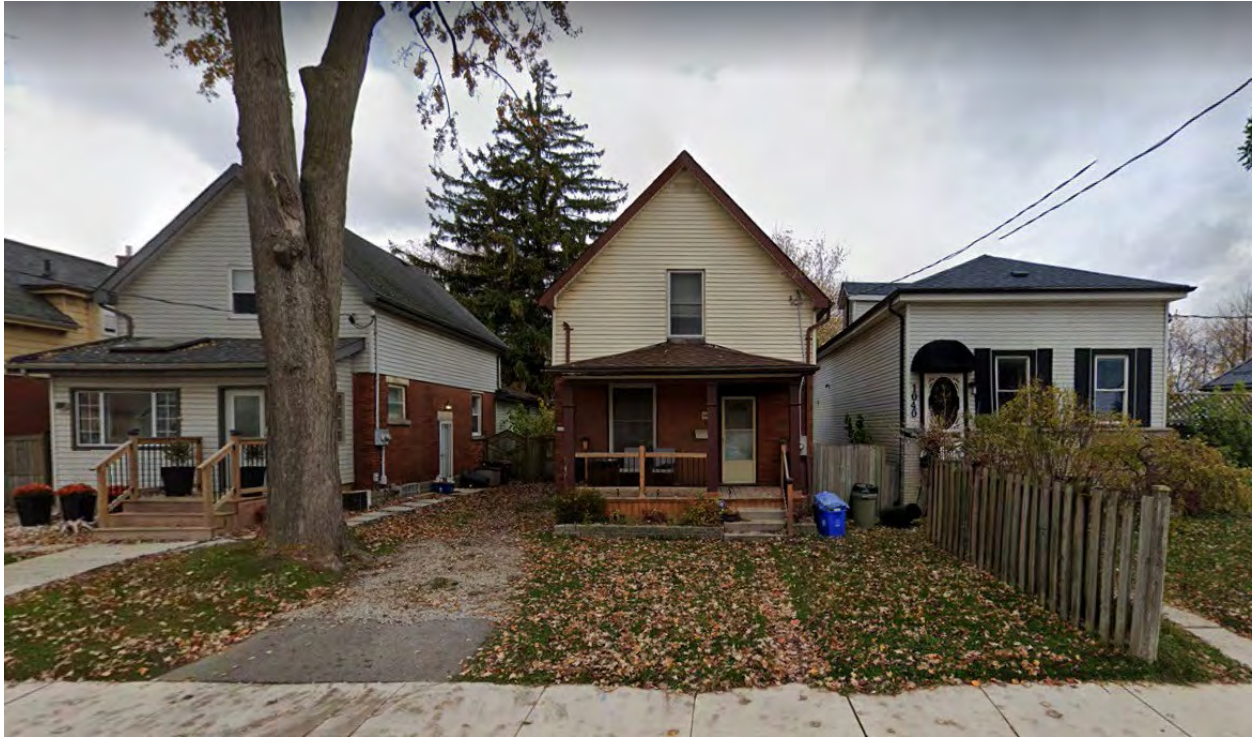
Image 5 - Low-density residential built form on King Street
