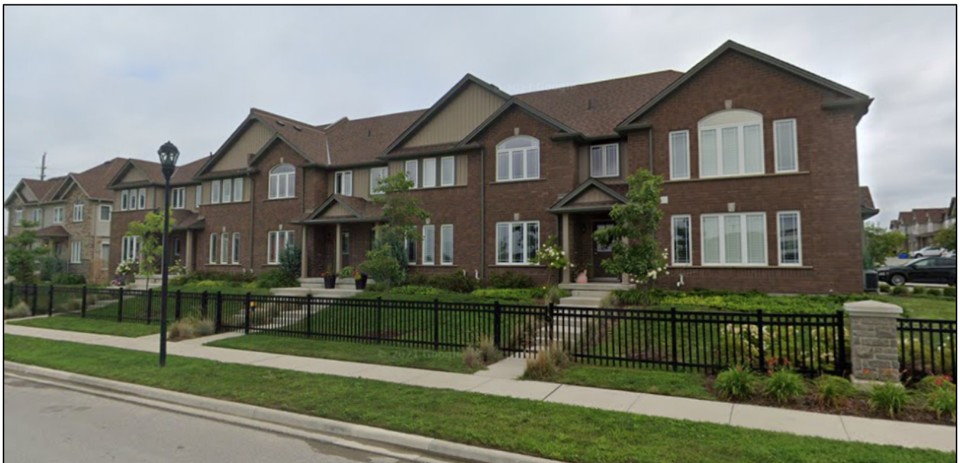
Photo 6. View of Medium Density Residential (Townhouses), looking east from Riverbend Road.
