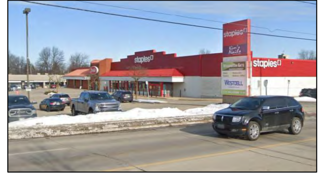
Photo 2. To the east of Subject Site, there is a strip commercial plaza, at 332 Wellington Road.
