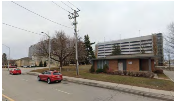
Photo 3. To the south of the Subject Site, there is a small hydro building and a large regional facility.
