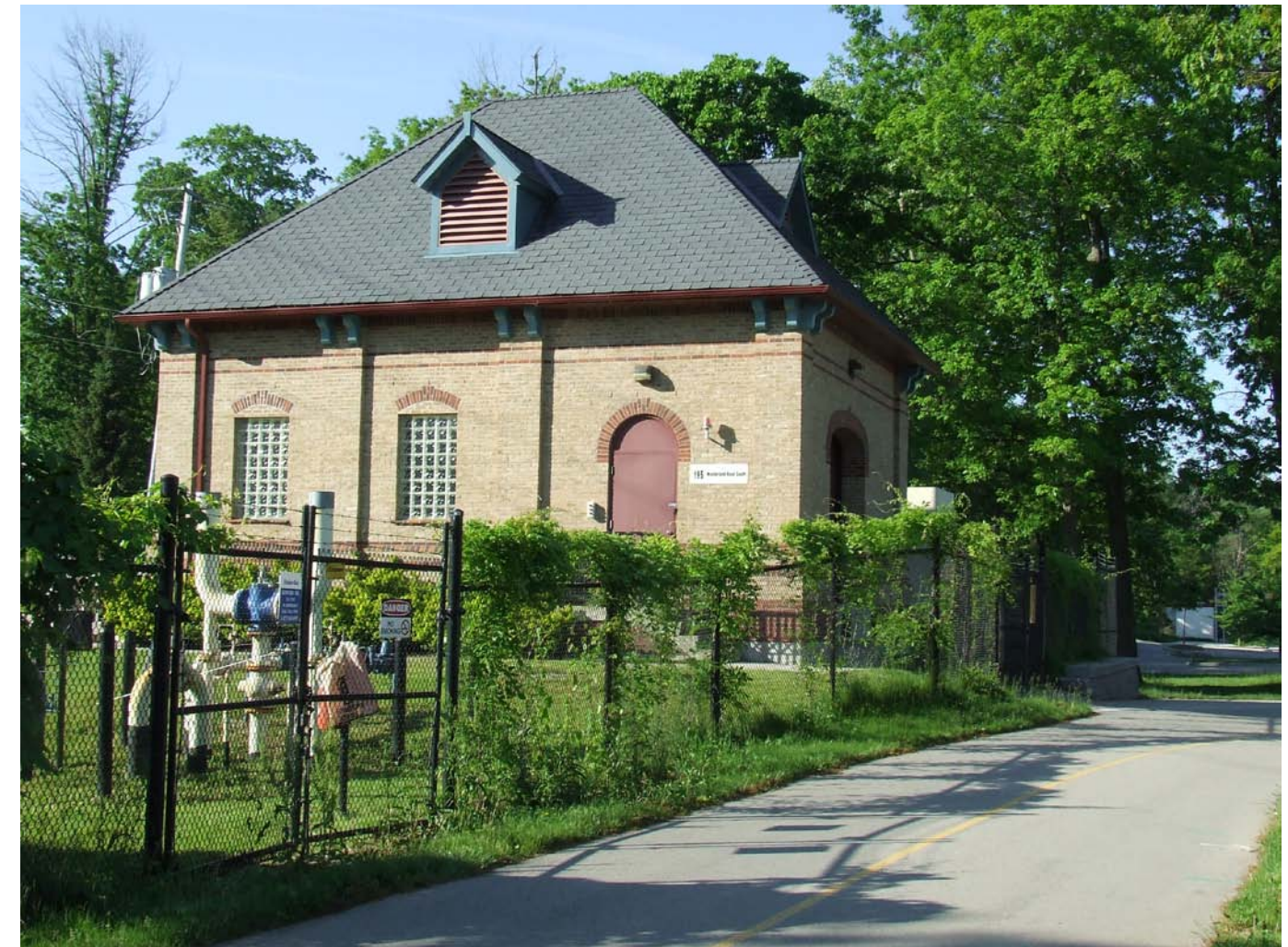
Municipal infrastructure in Springbank Park
